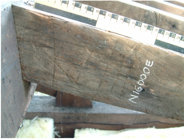
C: Race knife mark \diagdown\parallel\parallel on common rafter 6R8
