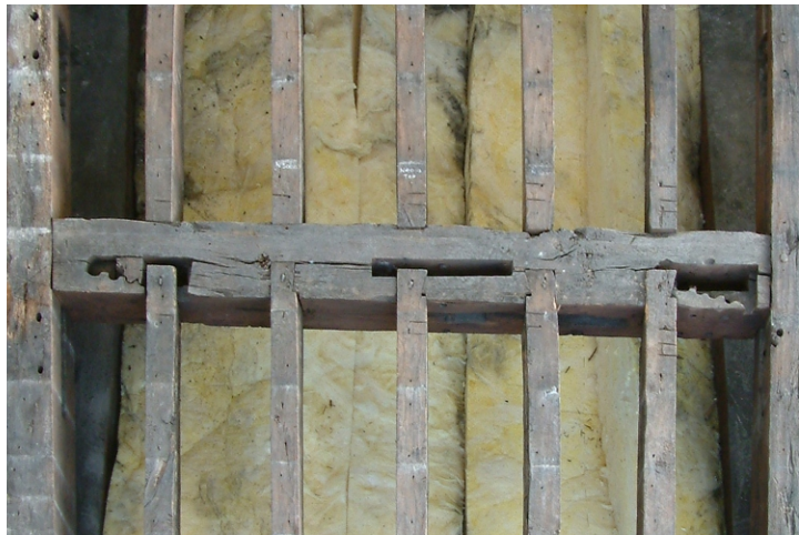
B: Group 2 timber reused as purlin P7 above compared to Group 1 timber reused as purlin P8 below
