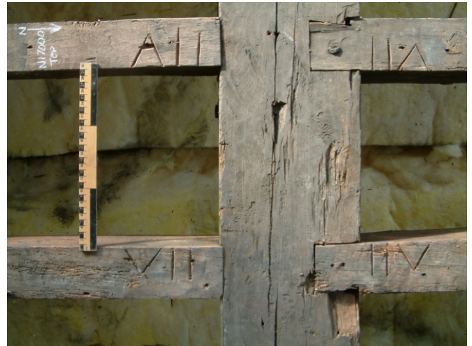
E: Common rafter marks in section 6 (6R7, 6R8 to left, 6R4, 6R3 to right)
