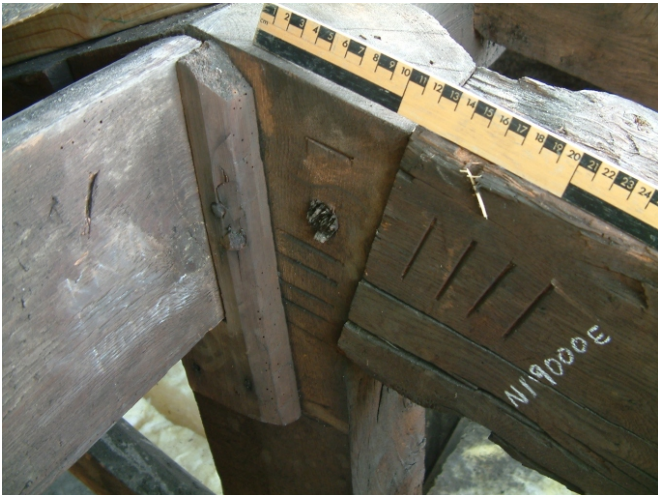
B: Marks where principal rafter PR4 meets king post KP4
