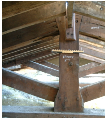
C: Trusses in the king post roof (KP2 at front)
