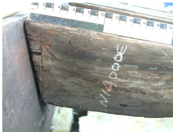
E: Truncated race knife mark \wedge on common rafter 6R10
