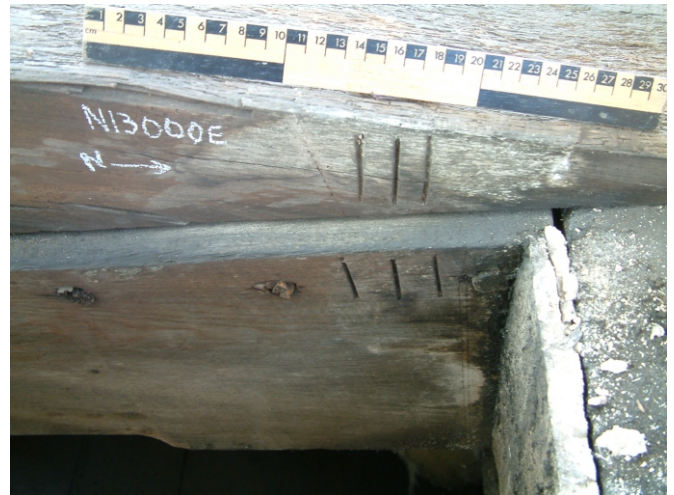
C: Marks where principal rafter PR3 meets tiebeam TB3
