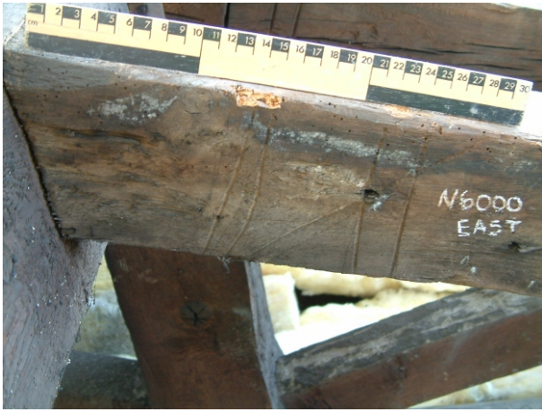
A: Race knife mark \parallel\parallel\parallel on common rafter 8R6
