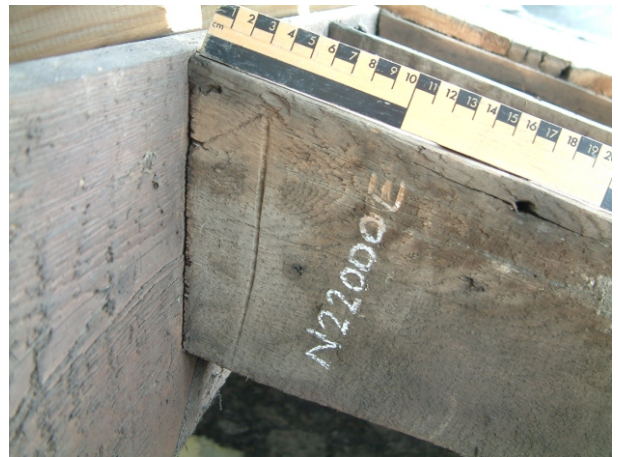
D: Race knife mark \uparrow on common rafter 5R7
