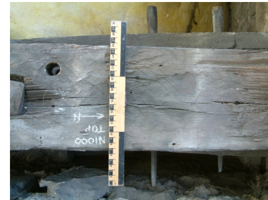
G: Intact draw pegs, points facing tower wall, indicating in situ truss construction (PR1 on Truss I)
