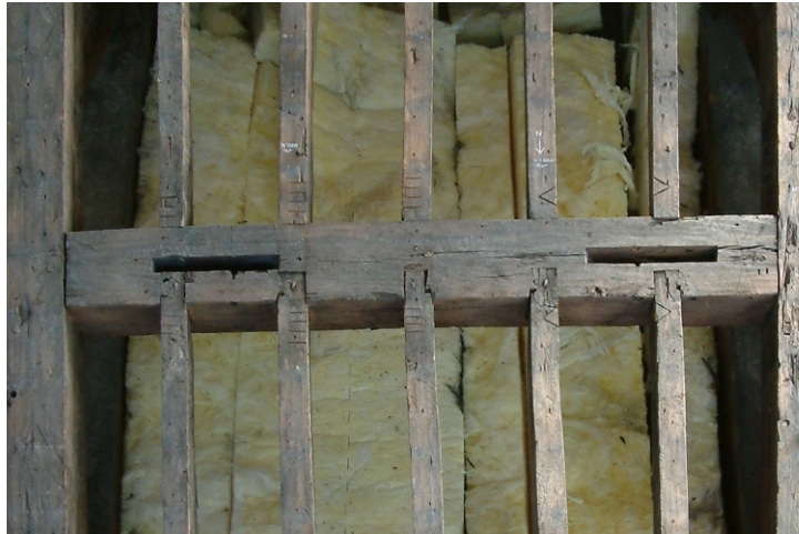
B: Group 2 timber reused as purlin P7 above compared to Group 1 timber reused as purlin P8 below
