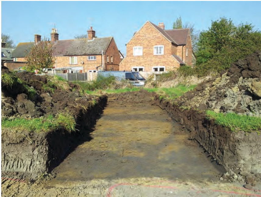
Figure 9. Photographs of Trench 5, looking South (above) and Trench 5 Extension (below)
