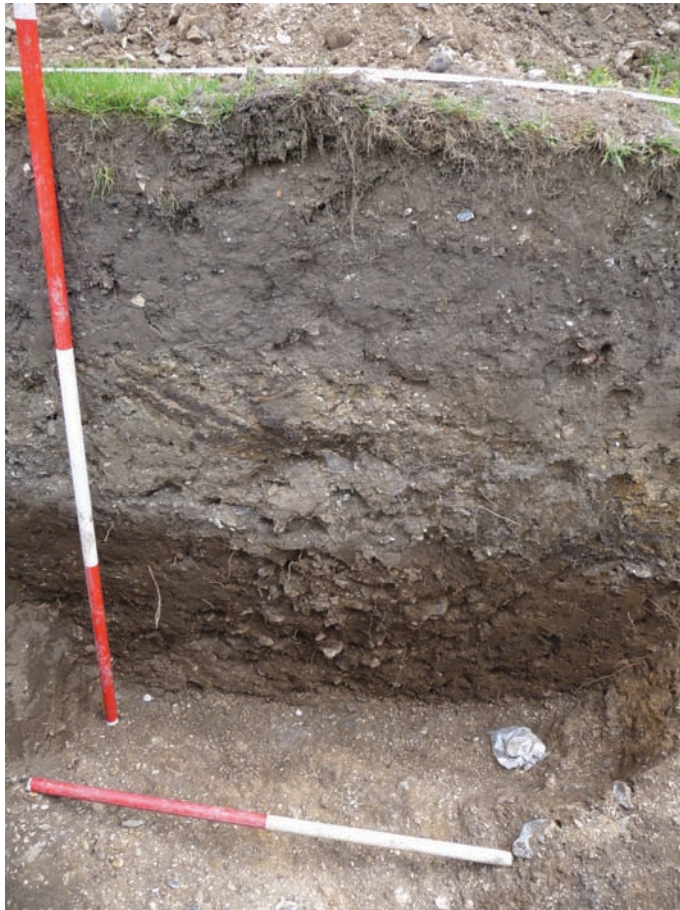
Figure 5. Photograph of ditch (F.1) cutting artefact-filled treethrow (F.2). West-facing section Trench 1.
