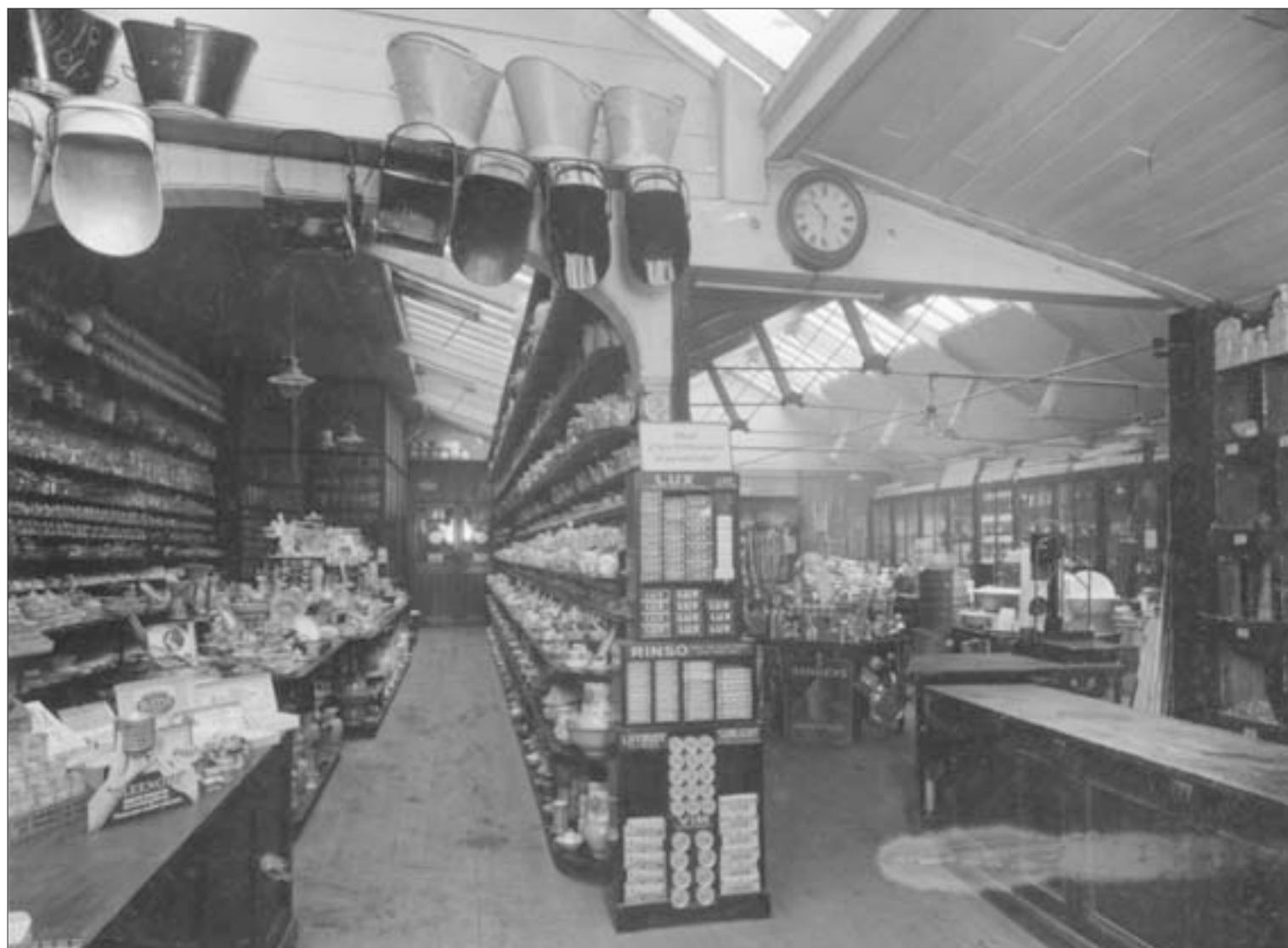
Looking West into Structures 96 (left) and 94 (right)
