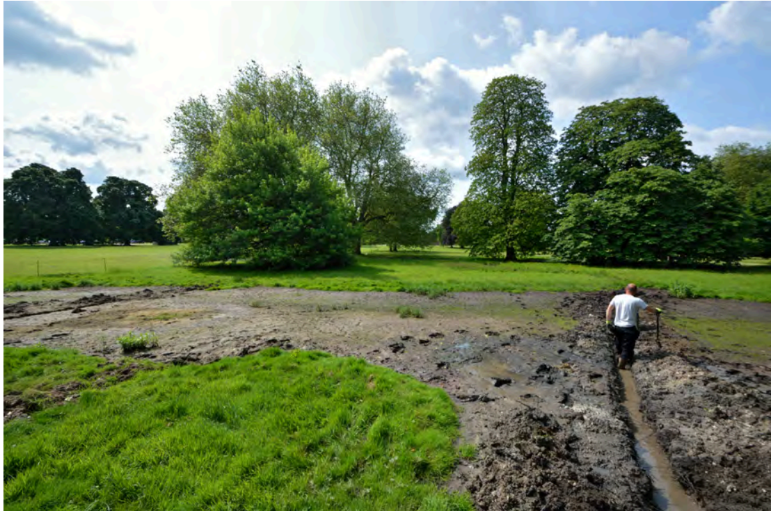
Figure 2: View of area of standing water looking south towards Audley End house. Source of leak is under trees to the right of the frame
