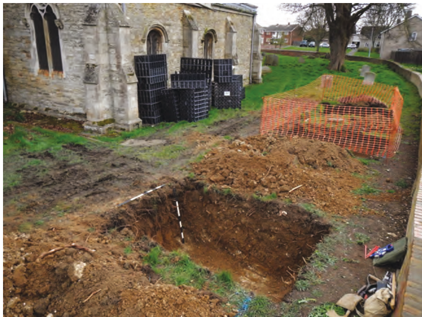
Figure 3. Soakaway 1 (top), Soakaway 2 (middle), and Soakaway 5, with 3 and 4 behind (bottom)
