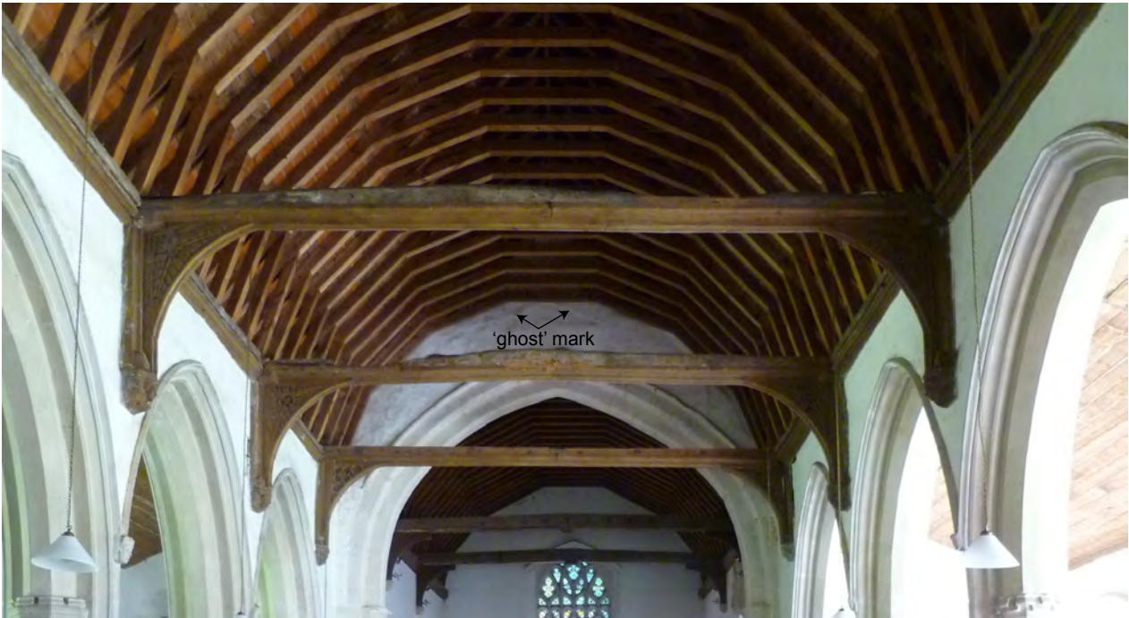
Tie Beams II, III and IV from Nave floor looking East
