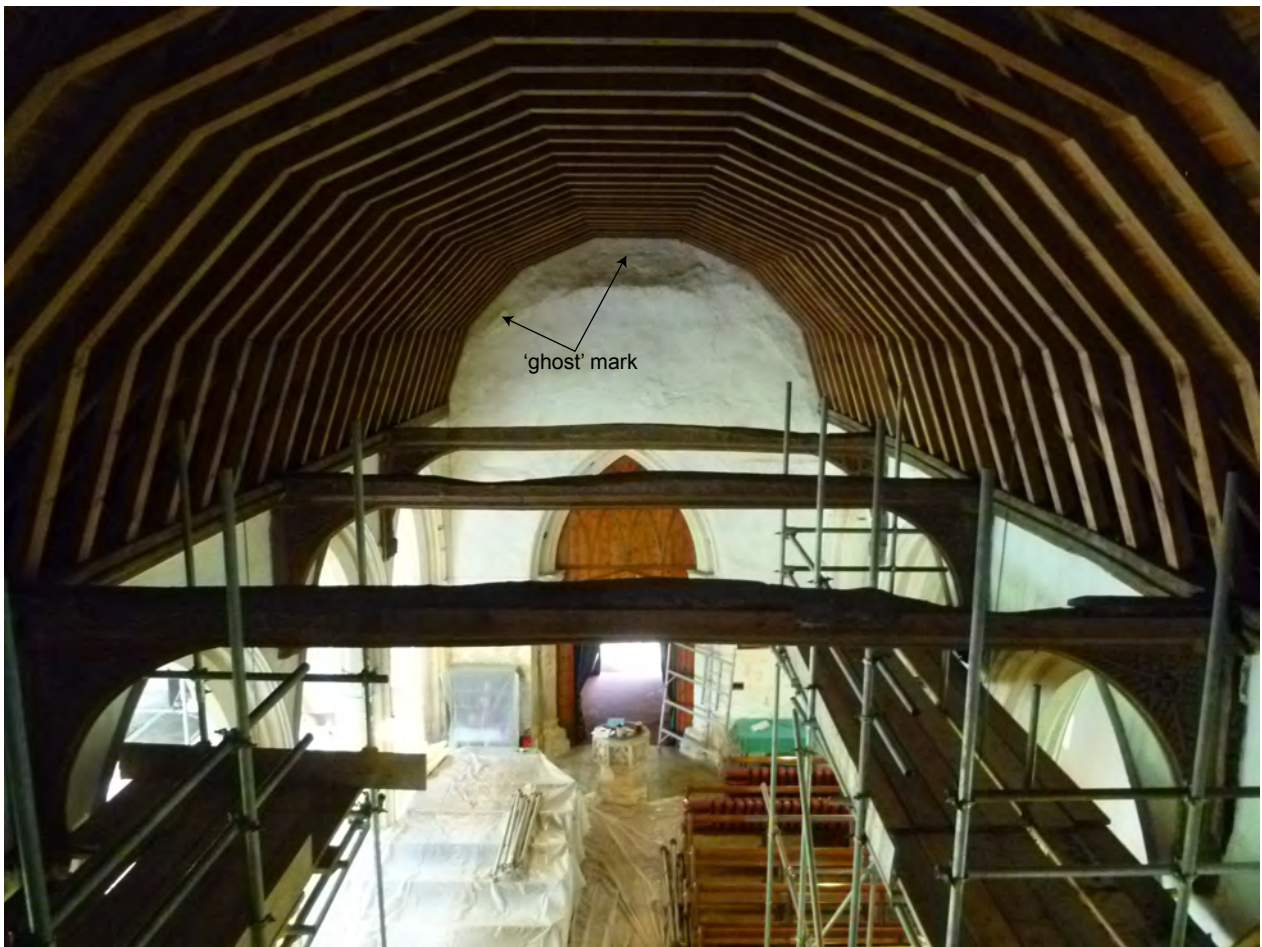
Tie Beams III, II and I looking West
