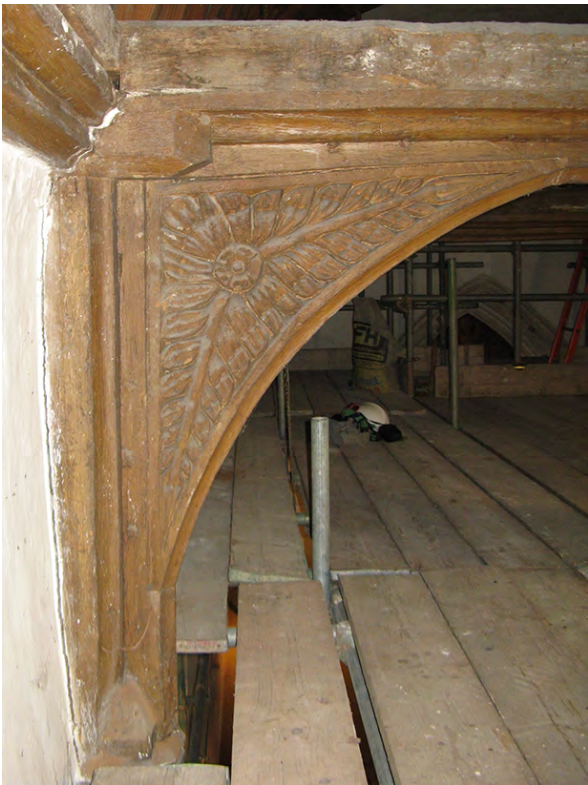
Tie Beam II southeast (design 3)
