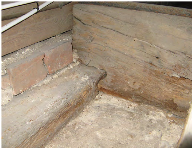
(c) Earlier outer wall plate tenoned to TBI
