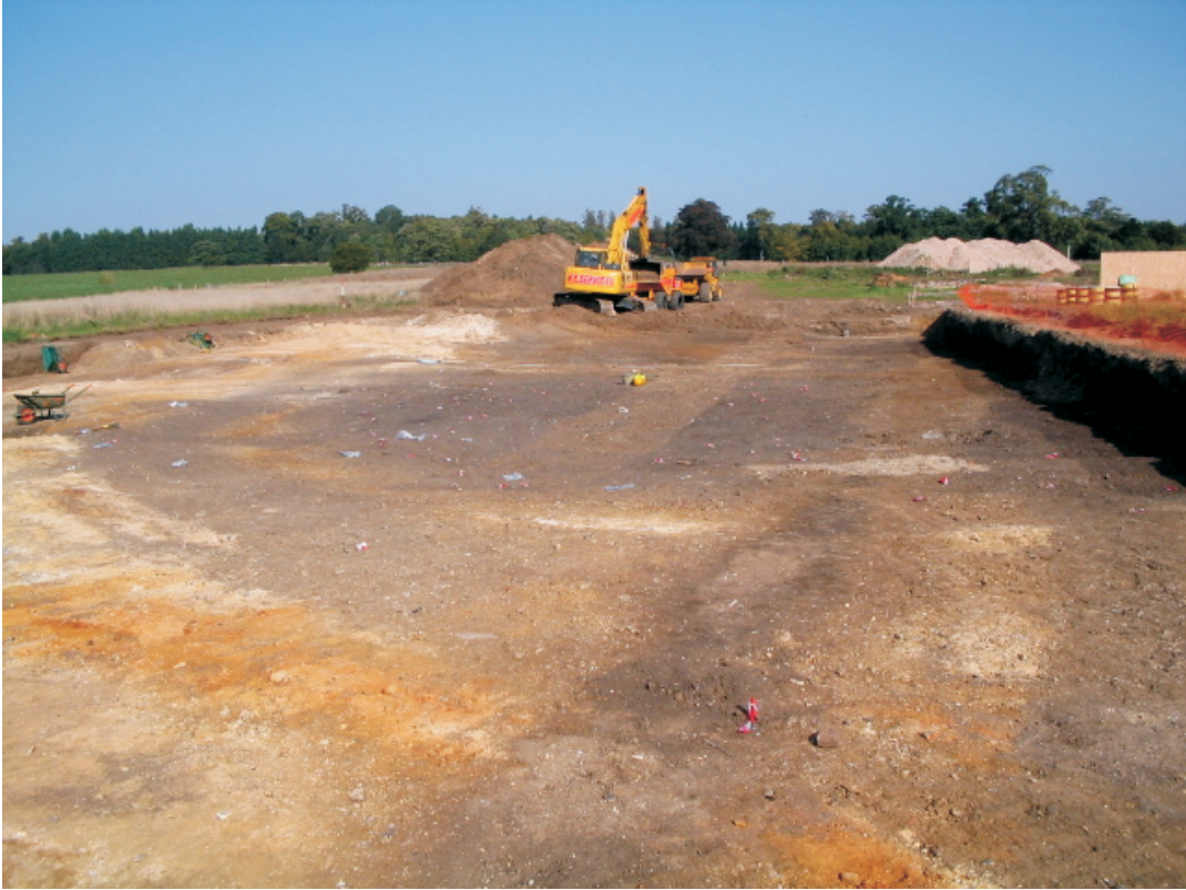
Figure 4. Photo of Hollow B looking north
