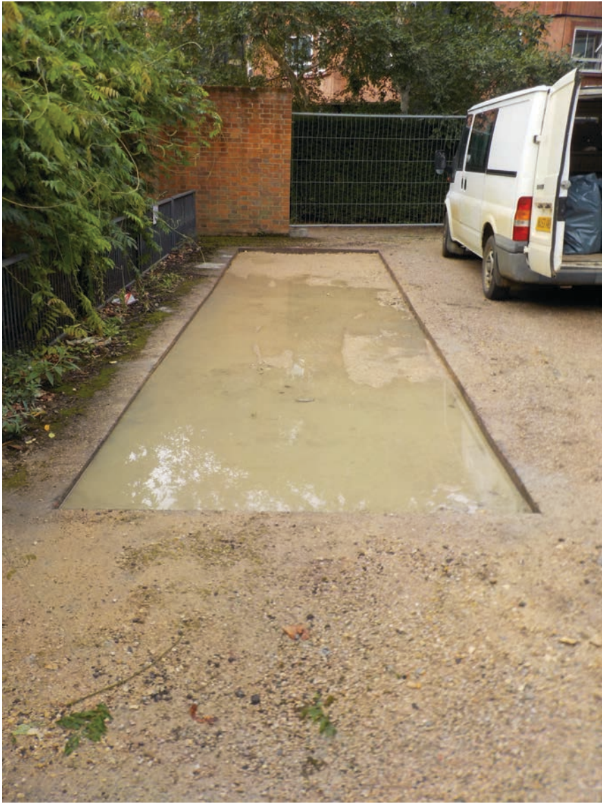
Plate 6. Trench 2, the concrete underlying the tarmac (looking South)
