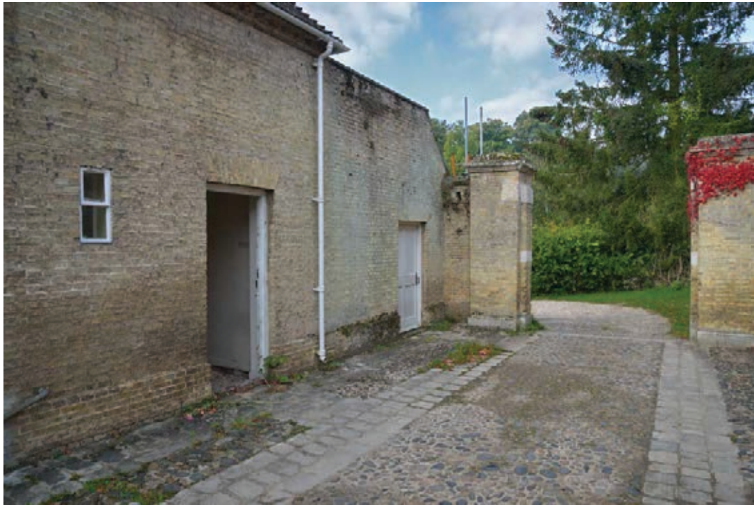
Figure 7. View of north facing west end of southern Stable Block
