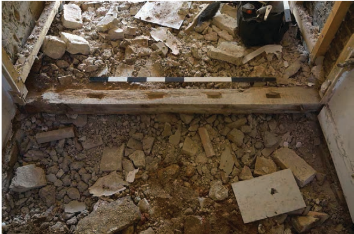
Figure 9. Wooden baseplate exposed in connecting corridor
