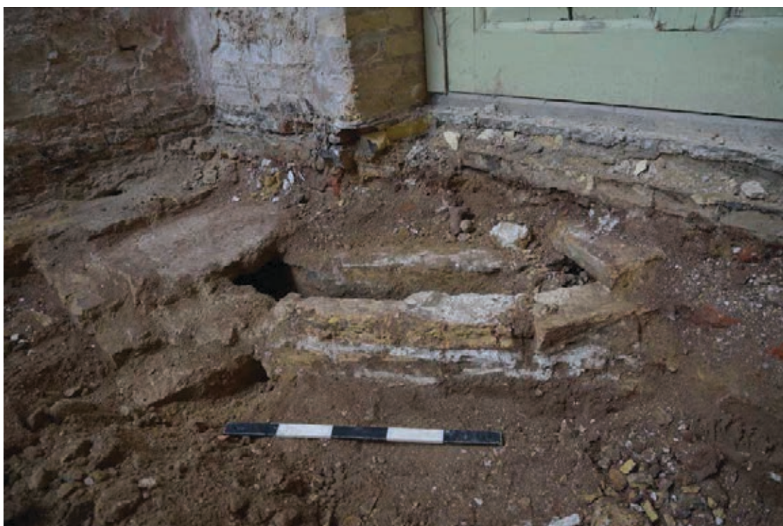
Figure 12. Drain serving soakaway in the north west corner of garage
