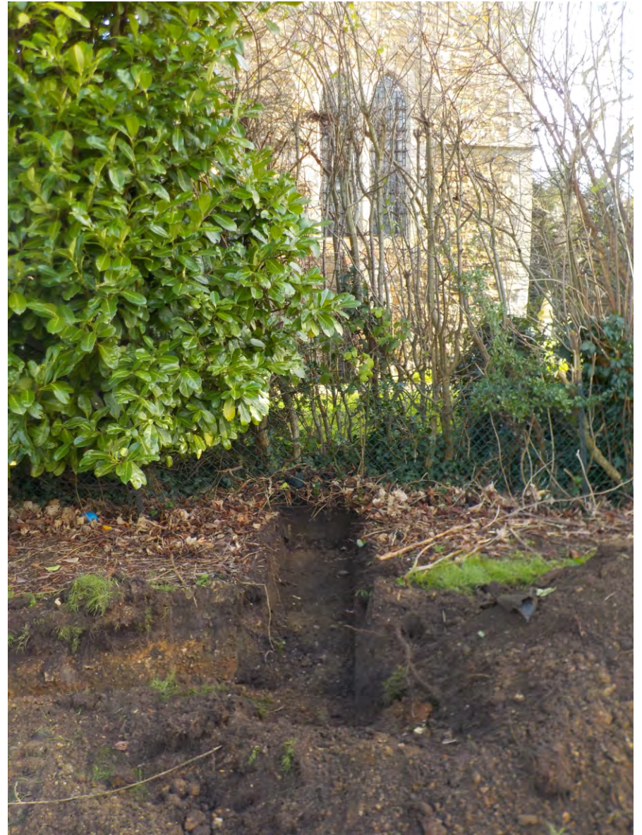
Plate 2. Trench turning east towards St Andrew's
