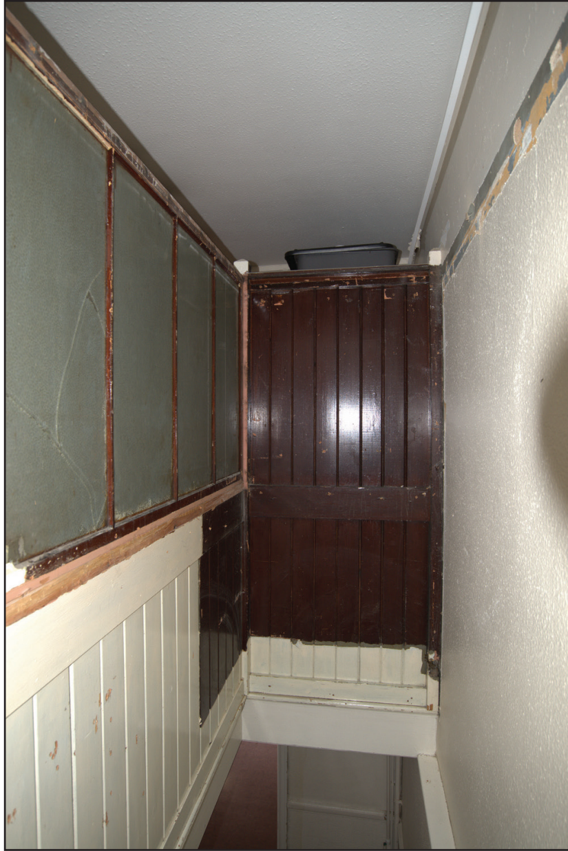
Figure 18. Details of the original panelling on the second floor. In No. 5, the formerly open balustrade has been extended to ceiling height (A), whereas in No. 7 it remains open but has a watertank installed above (B).
