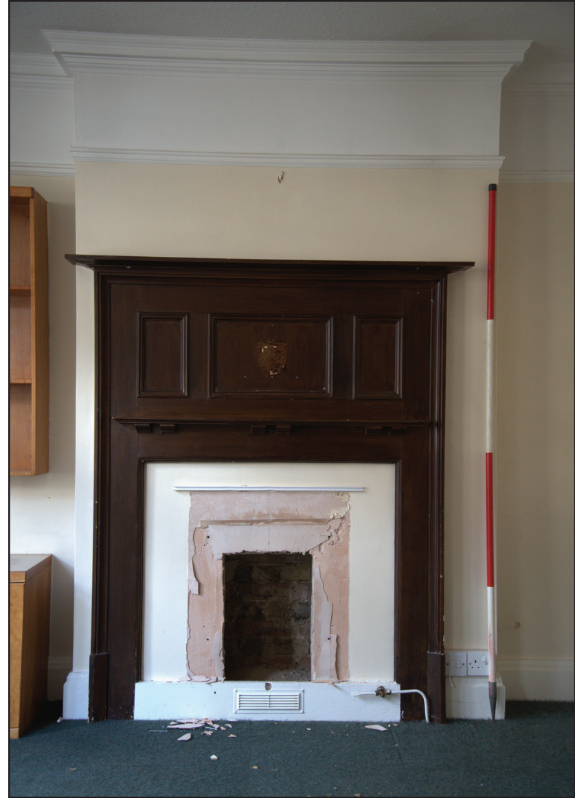
Figure 14. Detail of the fireplace in the rear parlour of No. 8 (A). The best preserved example in the terrace, this was the only remaining unblocked fireplace. The surround, which was also well-preserved, is different from those found in other properties, thereby providing a level of individuality. It is unclear whether the fires themselves varied to the same degree between houses; due to the cost involved, this appears less likely. In the master bedroom of No. 8 only the surround remains (B).
