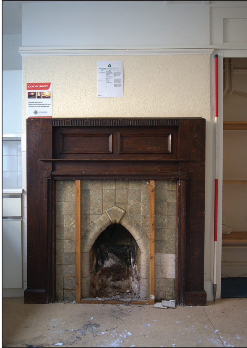
Figure 14. Detail of the fireplace in the rear parlour of No. 8 (A). The best preserved example in the terrace, this was the only remaining unblocked fireplace. The surround, which was also well-preserved, is different from those found in other properties, thereby providing a level of individuality. It is unclear whether the fires themselves varied to the same degree between houses; due to the cost involved, this appears less likely. In the master bedroom of No. 8 only the surround remains (B).
