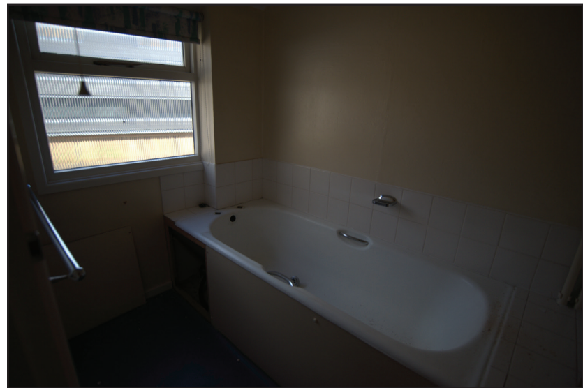
Figure 13. Views of the second storey, including the front bedroom of No. 7 (A) the rear bedroom of No. 8 (B) and the bathroom of No. 8 (C- formerly a linen closet?)
