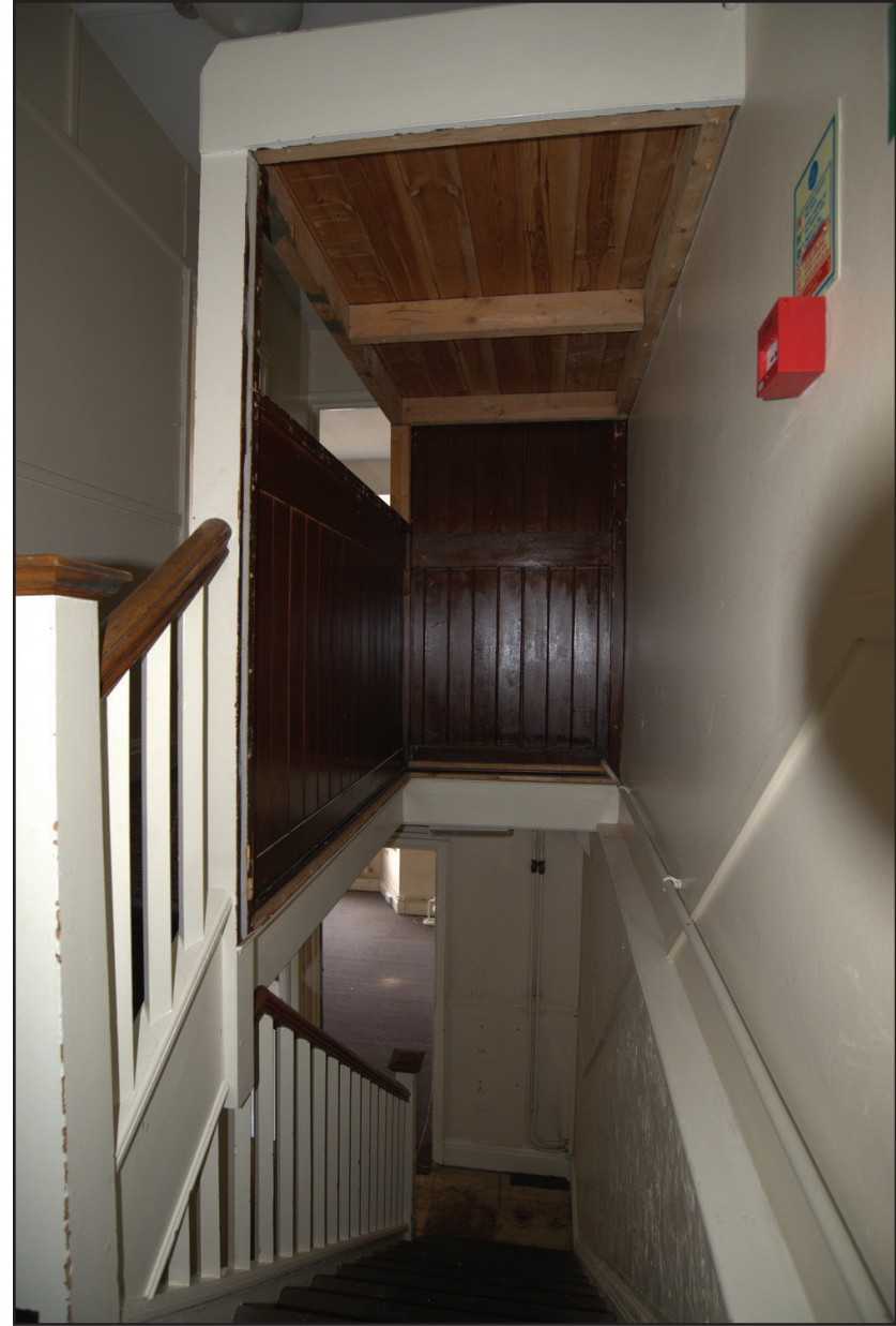
Figure 18. Details of the original panelling on the second floor. In No. 5, the formerly open balustrade has been extended to ceiling height (A), whereas in No. 7 it remains open but has a watertank installed above (B).
