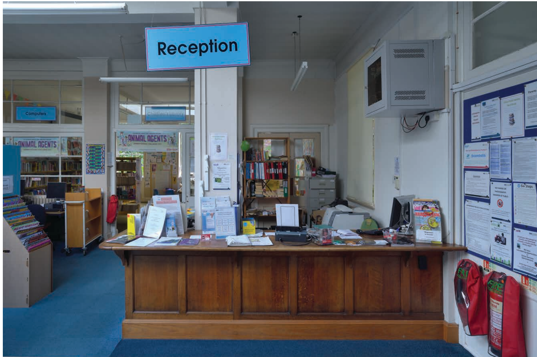
Figure 19. Detail of the reception desk, which employs elements reused from the original issue desk and perhaps also a reading table, facing southeast
