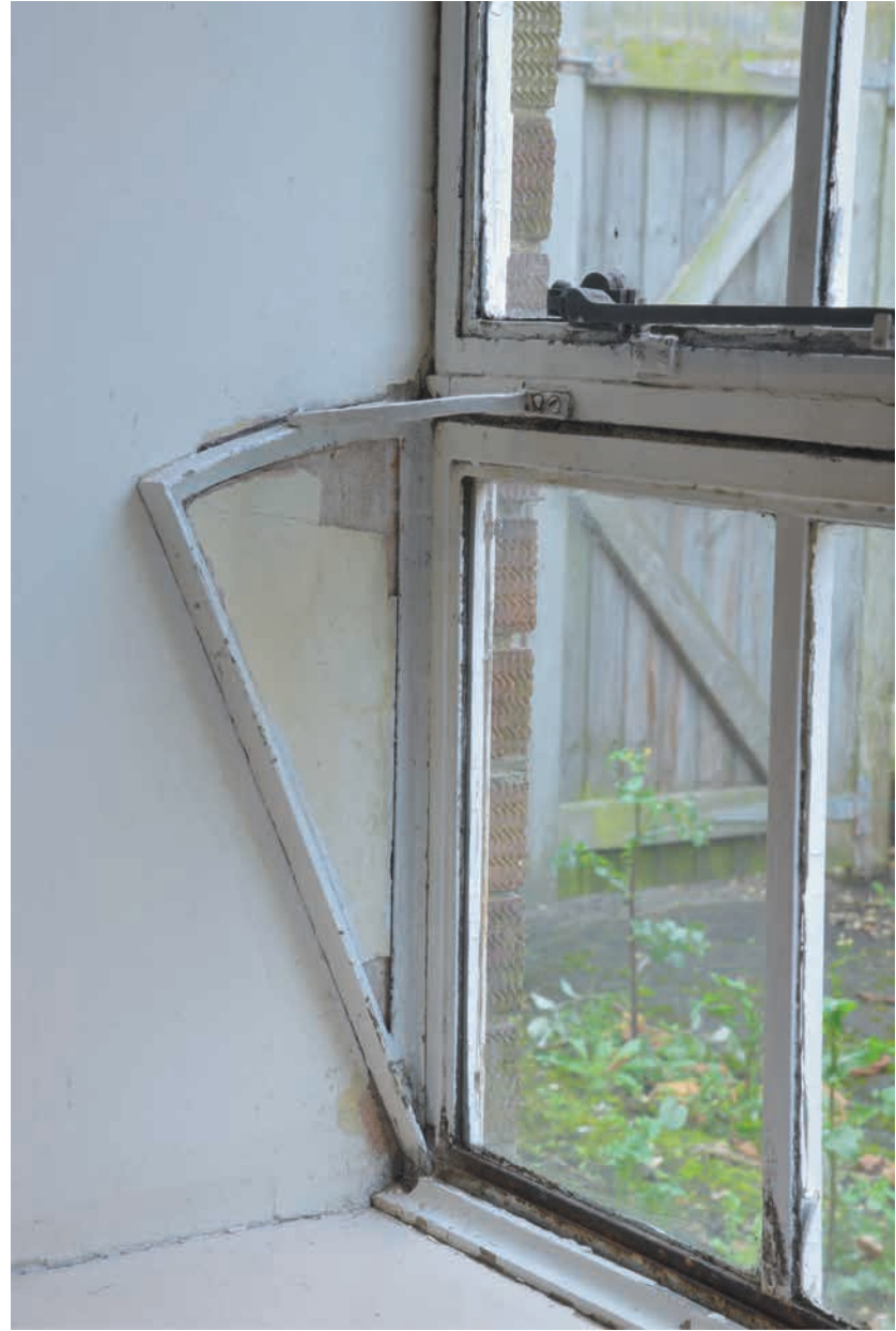
Figure 17. Details depicting a Crittall window in the Reading Room, facing northwest (left) and a close-up facing west (right)
