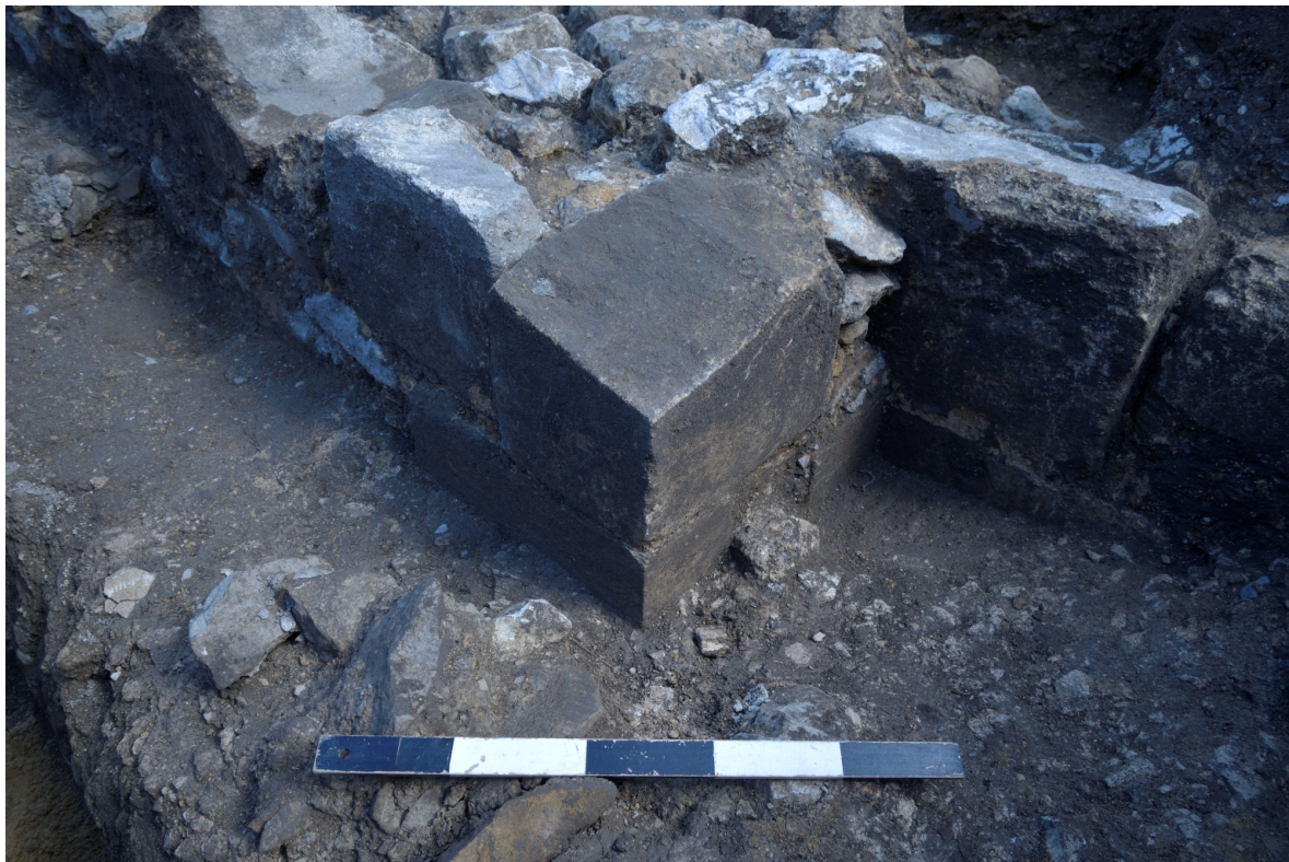
Figure 13. Photographs of the former chapel, showing; a fragment of the original flagstone floor and internal rendered walls (top, facing northwest) and ashlar quoining on the building's exterior southwest corner (bottom, facing northeast)
