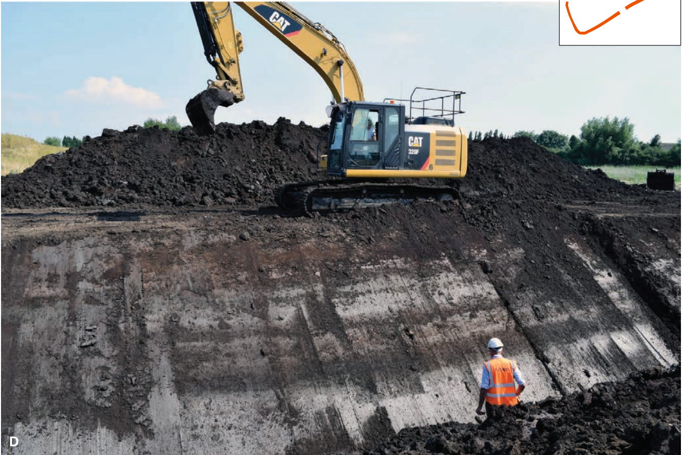
Figure 8. photographs of the monitoring of Drain Section C
