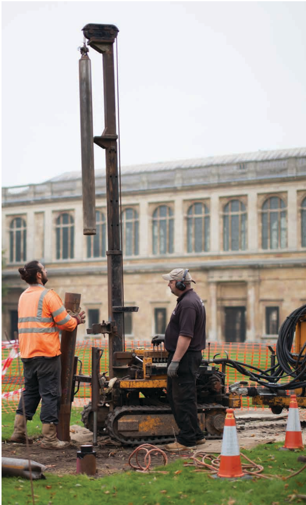
Figure 2. Photograph of boring in progress for concrete-piled foundation, facing northeast
