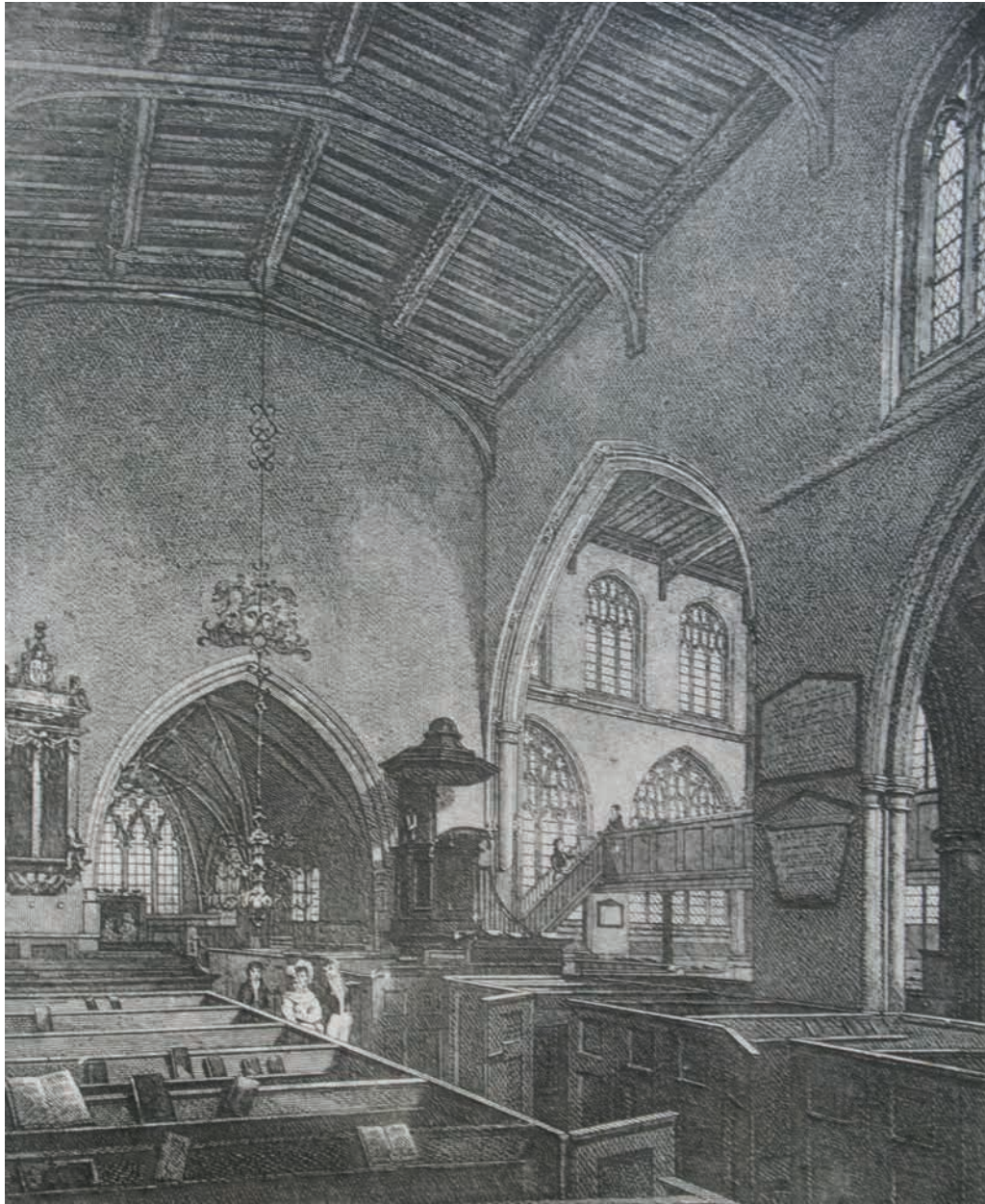
Figure 5. East-facing view of church's interior, c.1830, from Le Kleux's Memorials of Cambridge. This image depicts the nave and chancel prior to the extensive alterations that were undertaken in the 1830s
