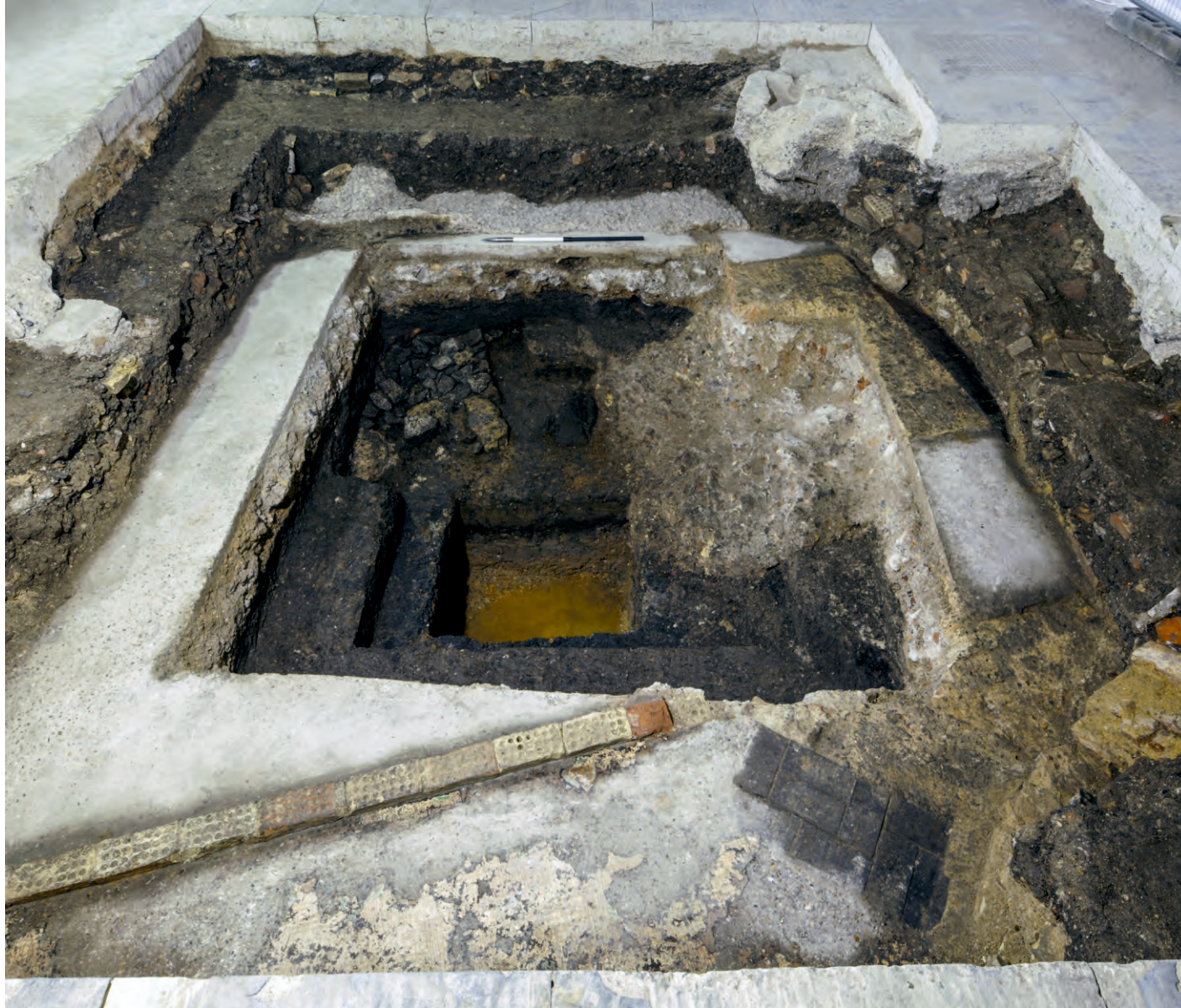
Figure 15. View of Trench 3, facing southeast, following the completion of excavation. Note the depth of the mortared rubble foundation of the Victorian building, including a substantial chimney base. Nevertheless, a significant sequence of Roman and pre-Roman deposits survived beneath this truncation
