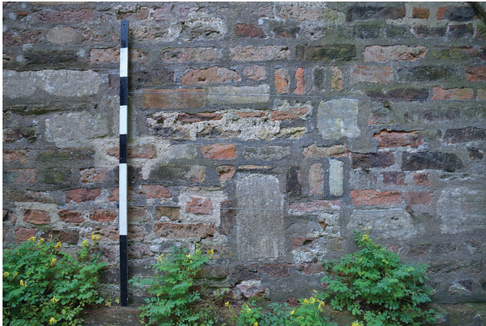
Figure 4. Photographic survey of the west-facing elevation of the west Chimney wall, with inset details showing extensive use of reused masonry and repeated episodes of repair and repointing undertaken to the fabric
