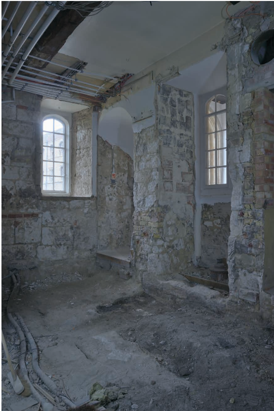
Figure 9. Photograph facing northeast within the Porter's Lodge, showing the flat-laid peg tile utilised in facing the window embrasure in the east wall and a portion of the masonry footing for the original eastern staircase exposed below floor level
