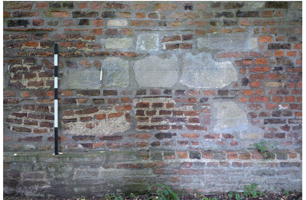
Figure 4. Photographic survey of the west-facing elevation of the west Chimney wall, with inset details showing extensive use of reused masonry and repeated episodes of repair and repointing undertaken to the fabric
