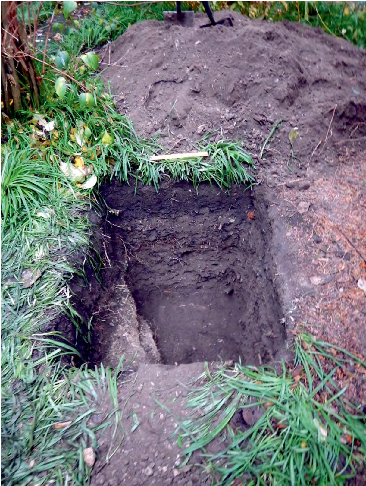
Figure 5. View of Trial Pit 3, facing southeast
