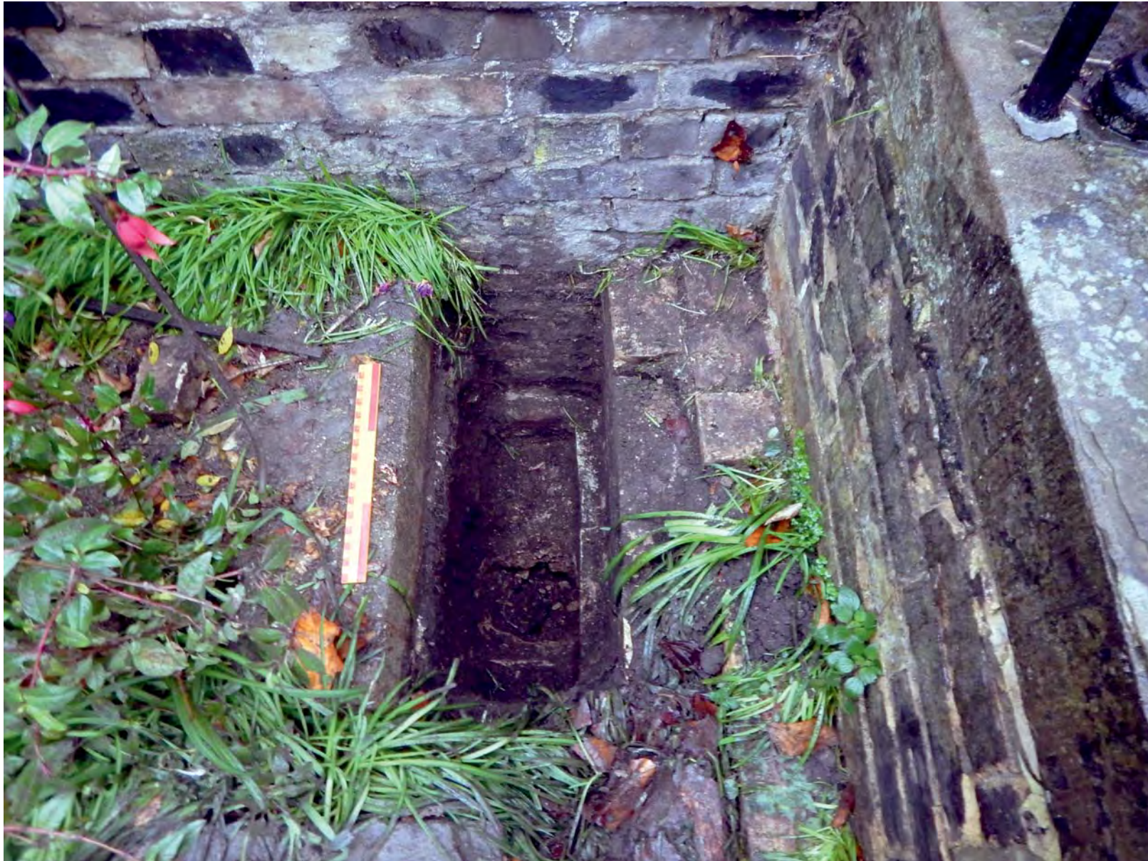
Figure 3. View of Trial Pit 1, facing northwest
