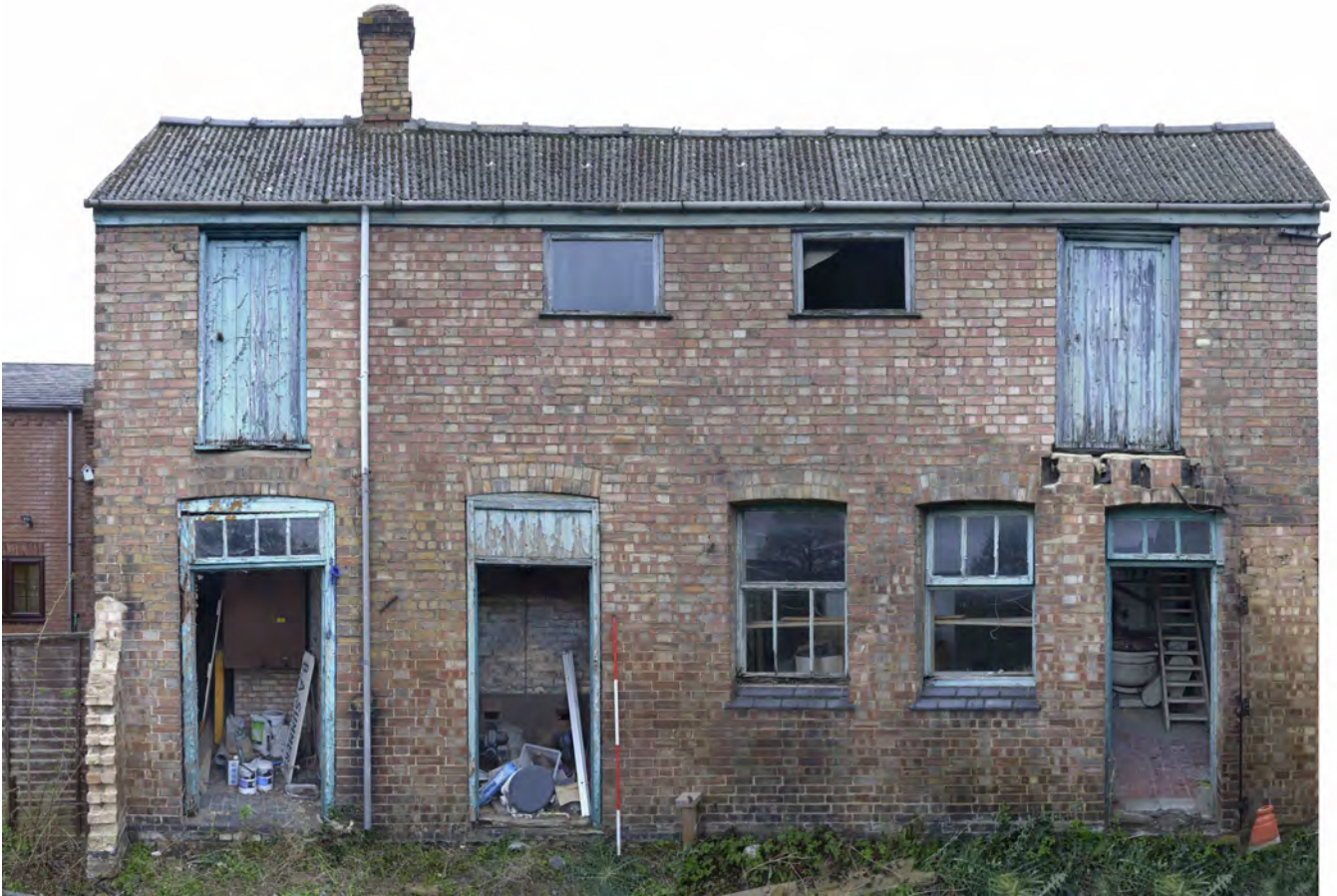
Figure 8: West elevation of bakery building ( composite image )
