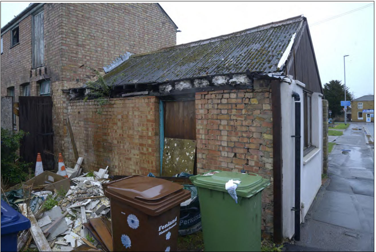
Figure 10: West wall of shop
