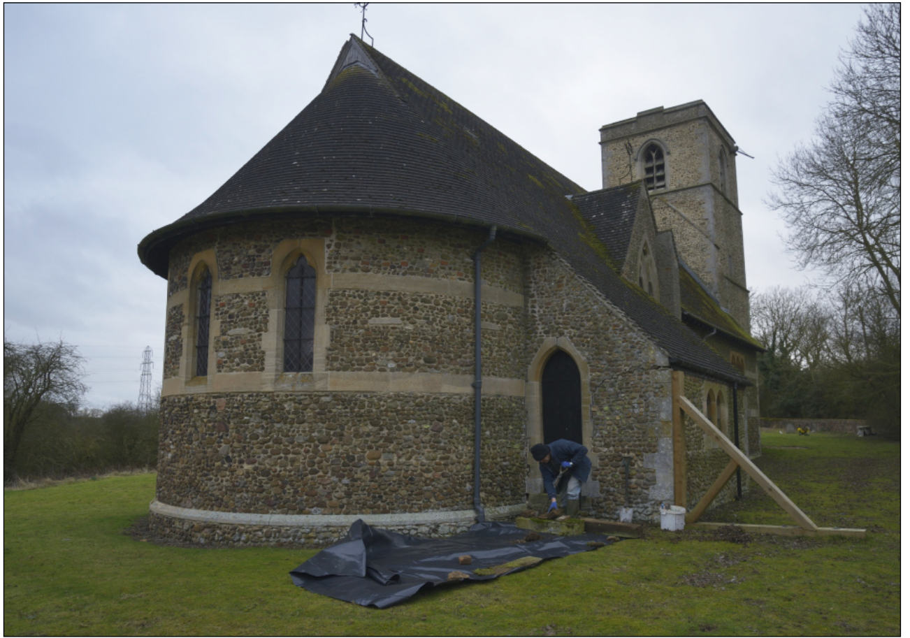
Figure 3: Apsidal West End of Church
