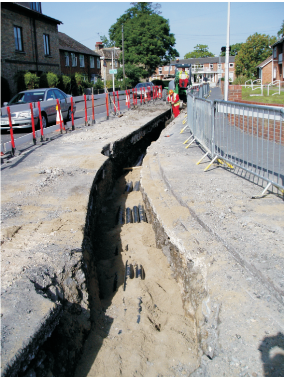
Zone 3: Water Lane
