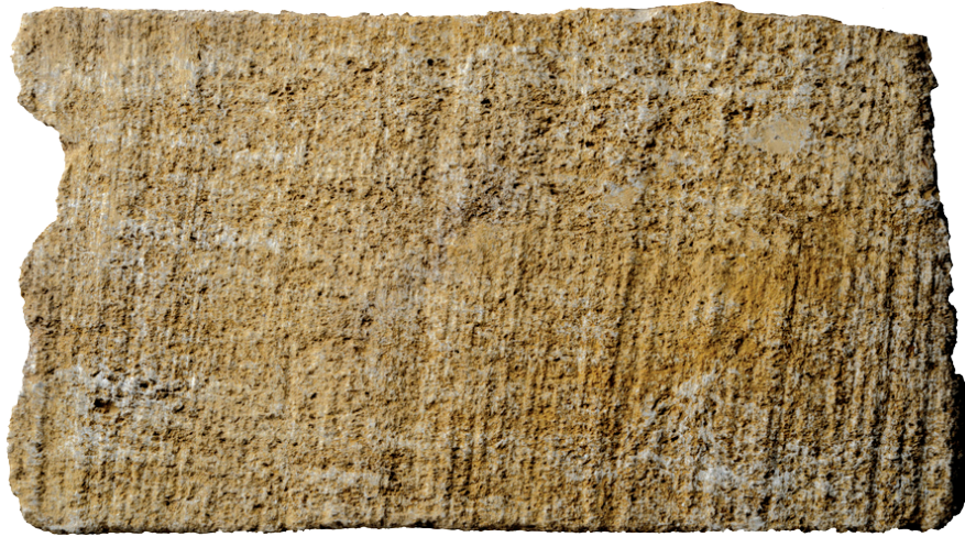
b) Saw cut stone
