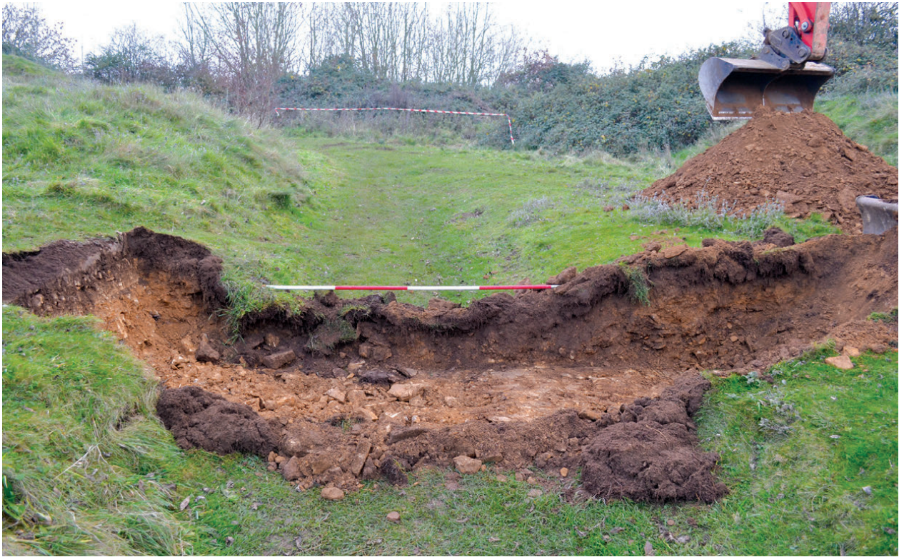
a) Tr. 7 - trench through trackway earthwork
