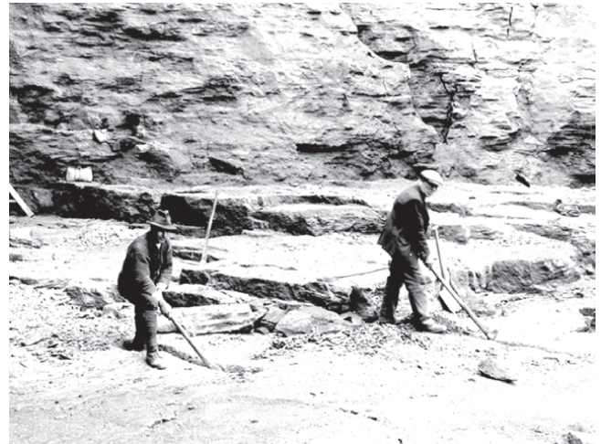
c) Slab excavation at Ham Hill in 1922 by J.Rhodes
