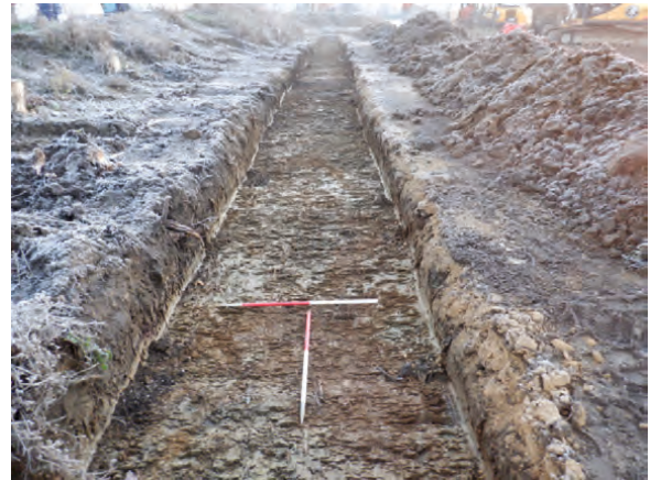
Tr.21 looking east
