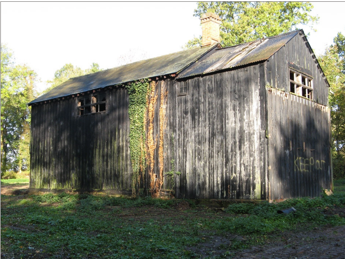
Figure 4: The Toilyard Building from the south east
