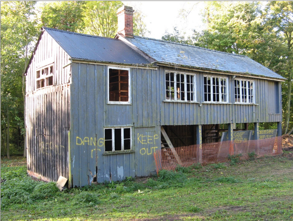
Figure 3: The Toilyard Building from the northeast
