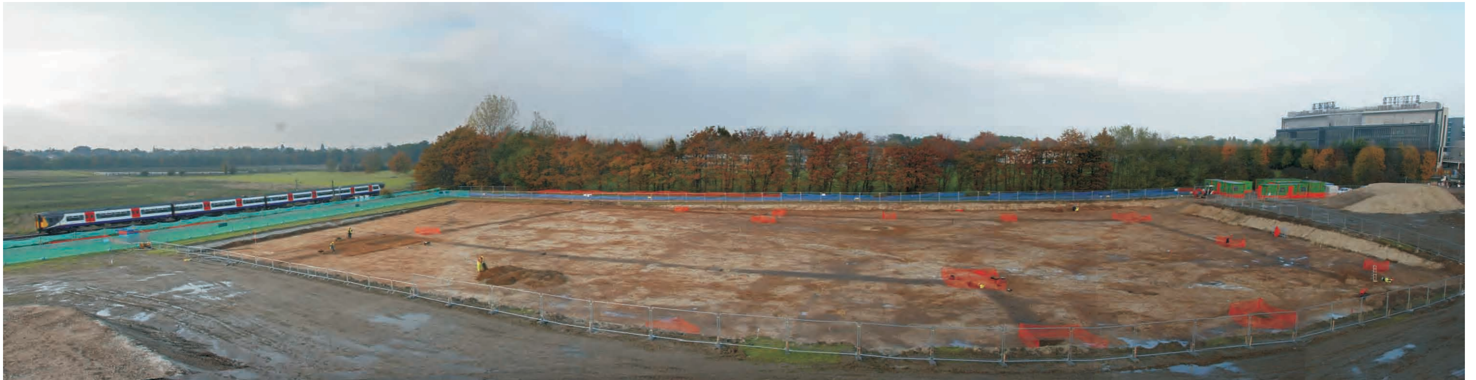
Figure 10. The site under excavation, showing the enclosure system.
