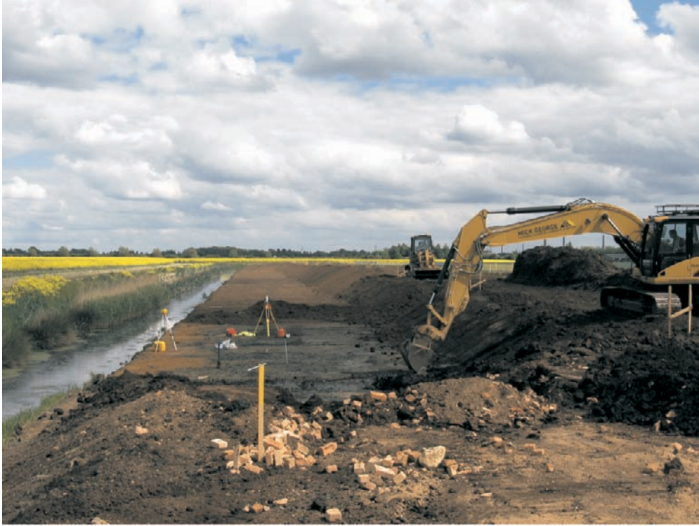
Figure 2. Photograph of widening of Padholme Drain (Site 1)
