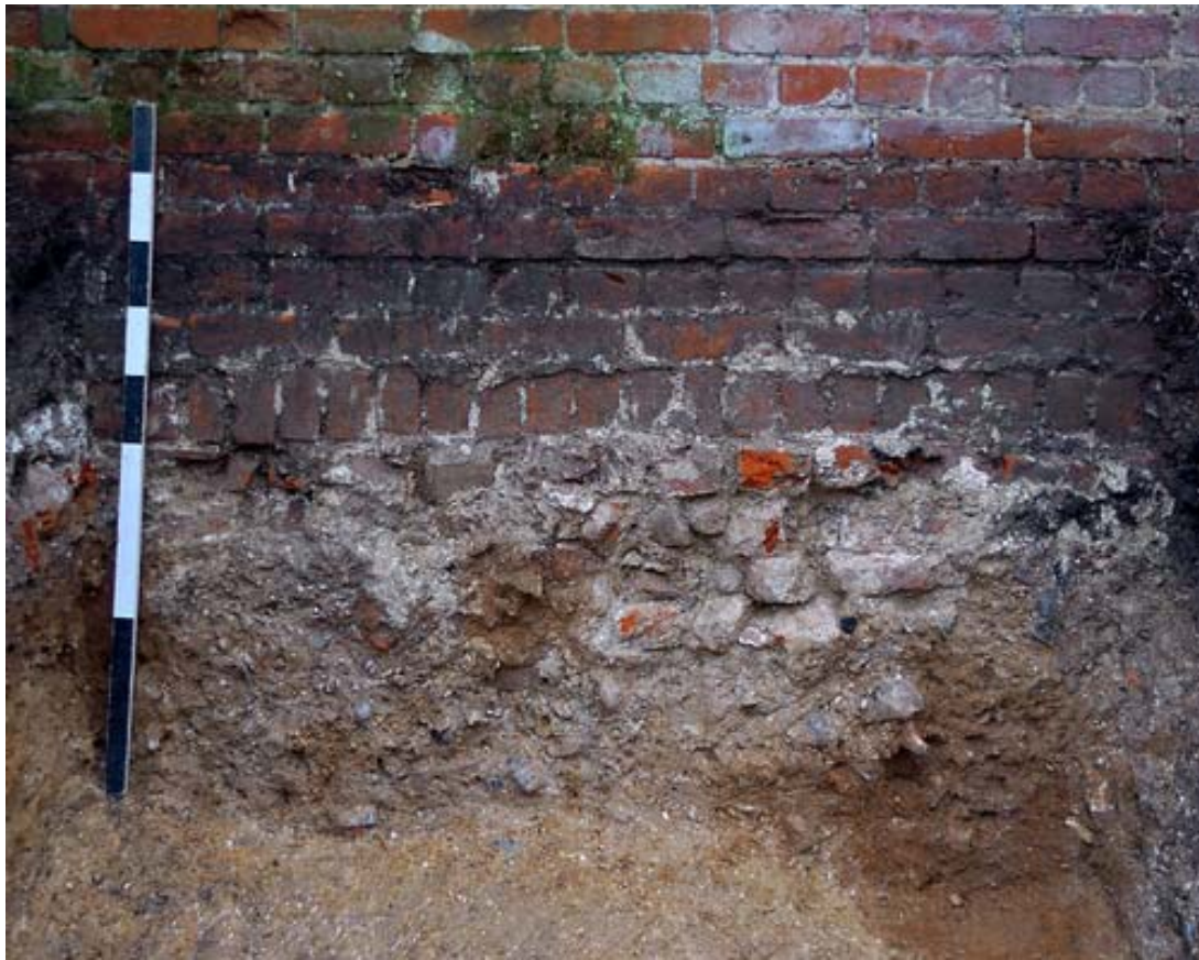
a) North facing section of Coach House wall.
