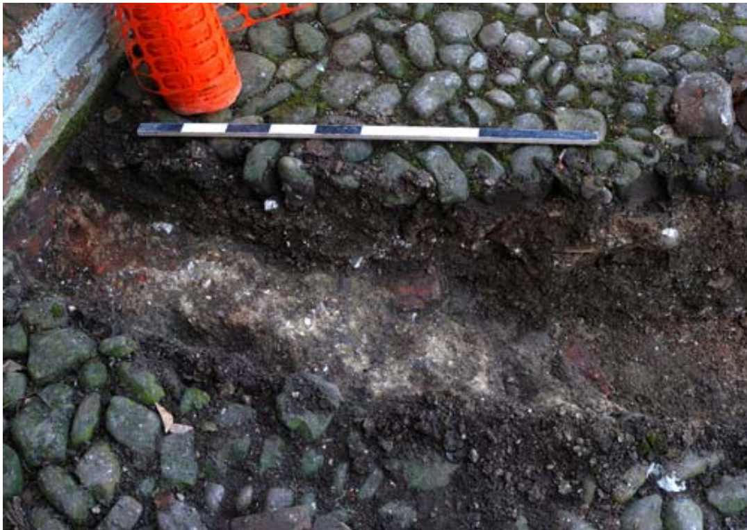
b).Mortar Spread in front of Stable Block
