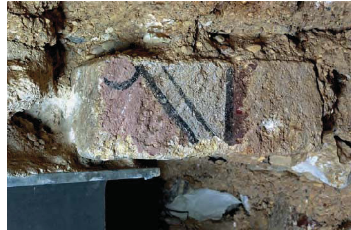
Figure 7: Doorway in north wall of Chapel prior to unblocking, with capital fragment (top right) and painted ashlar (bottom right) used in infill.
