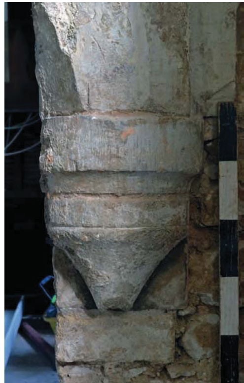
Figure 14: Details of capitals carrying chapter house vault (north pier bottom right, remainder central pier).
