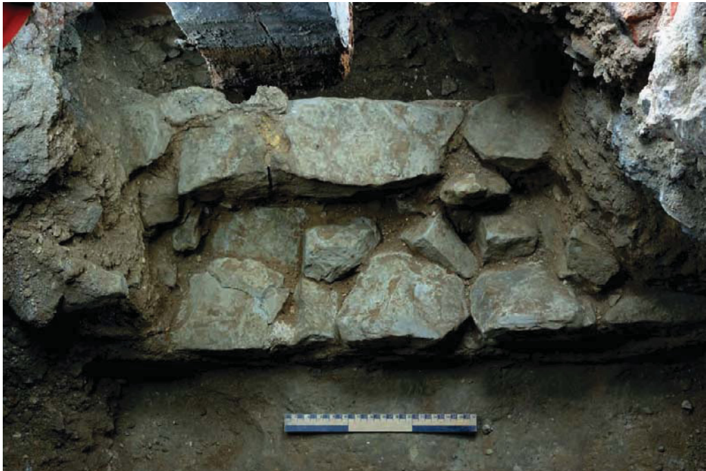
Figure 4: Detail of in-situ wall shaft F.46 (above), and later dividing wall F.47 (below).
