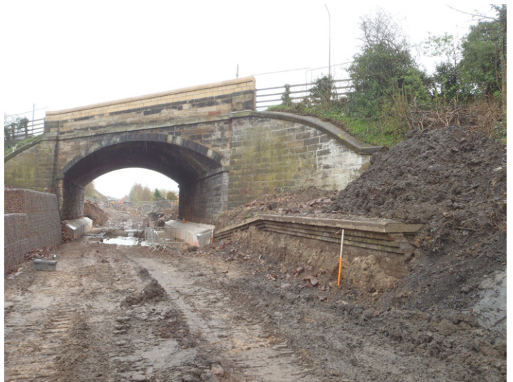
Fig. 8 - Stripping of western platform at Site 85 (Newtongrange Station)
