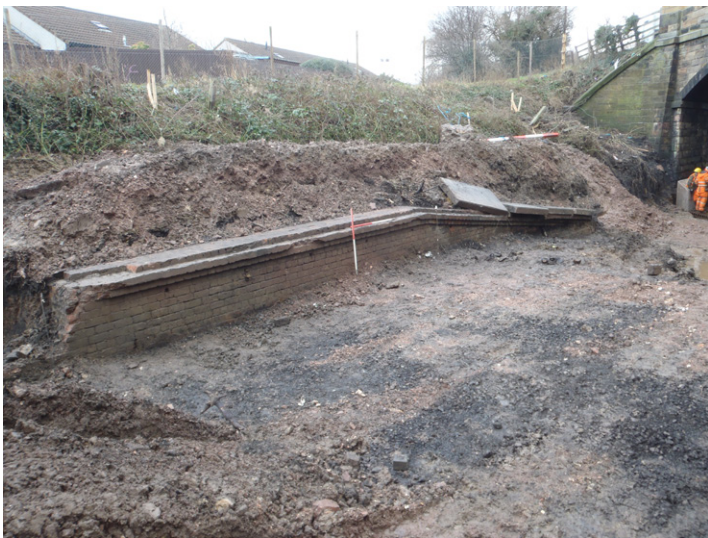
Fig. 7 - Stripping of eastern platform at Site 85 (Newtongrange Station)
