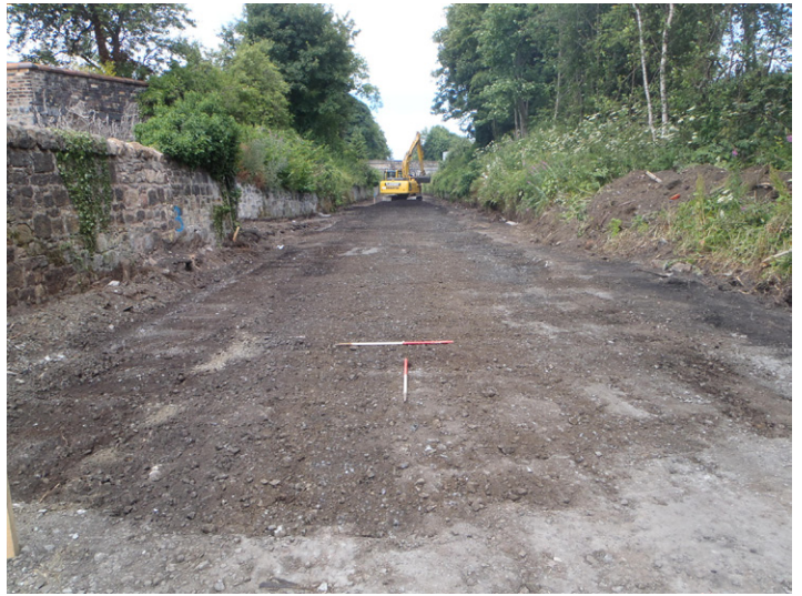
Fig. 6 - Stripping of track bed at Site 58 & 59 (Hardengreen junction)
