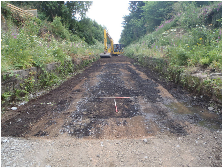
Fig. 5 - Stripping of track bed at Site 51 (Eskbank and Dalkeith Station)
