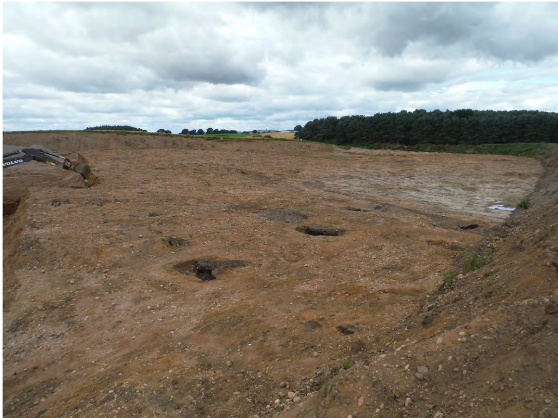
Fig. 3 General shot of Phase 4 Stage 2
