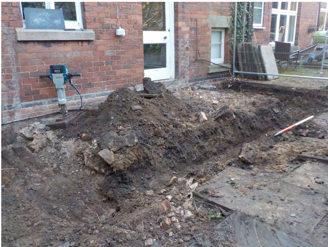
Fig. 2.2 Excavated foundation trench, facing south-west
