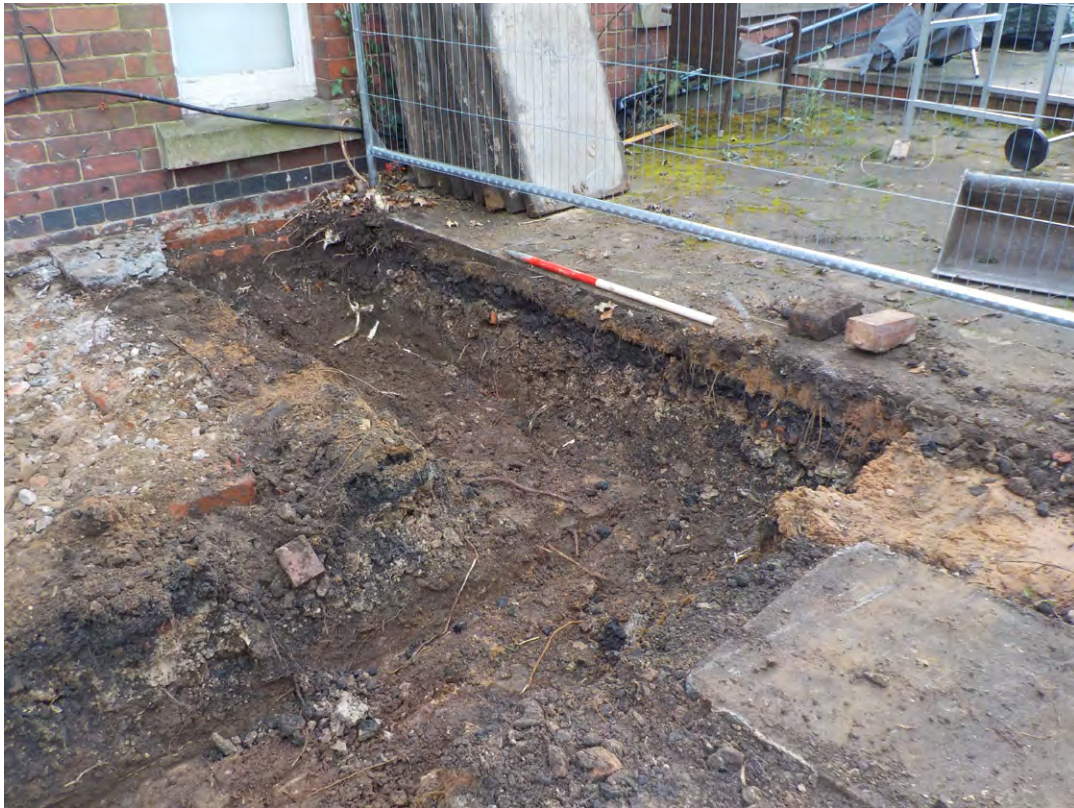
Fig. 2.1 Sample section of trench, facing south-west
