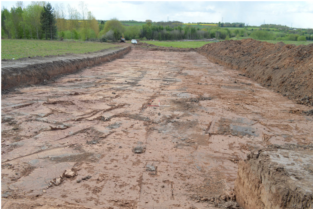
Fig. 2.2 - General post excavation shot looking south
