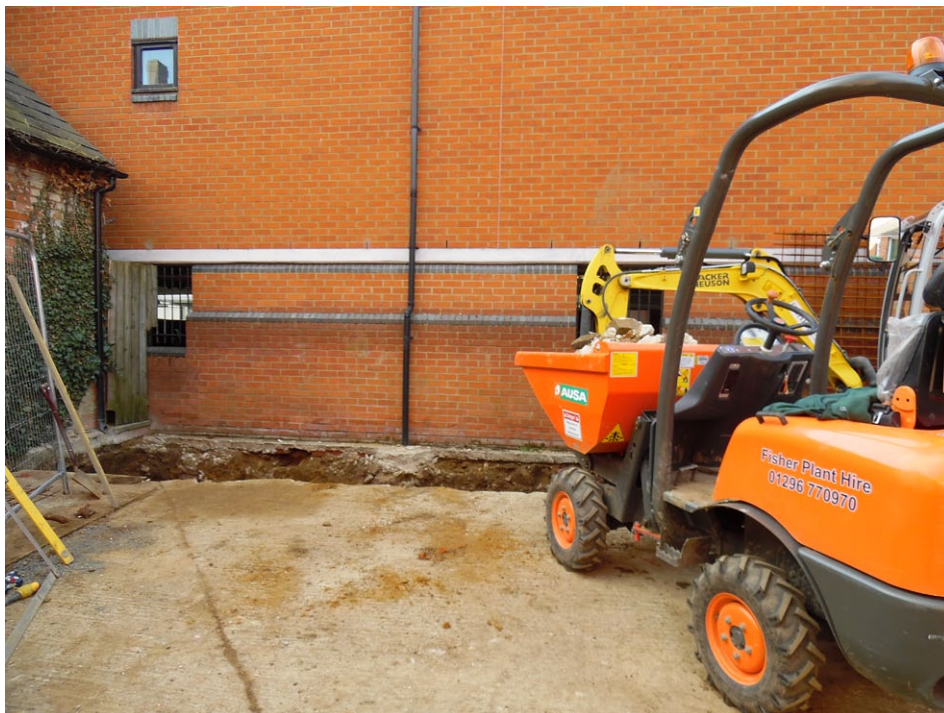
Fig. 4 - General shot of Site, taken from the N
