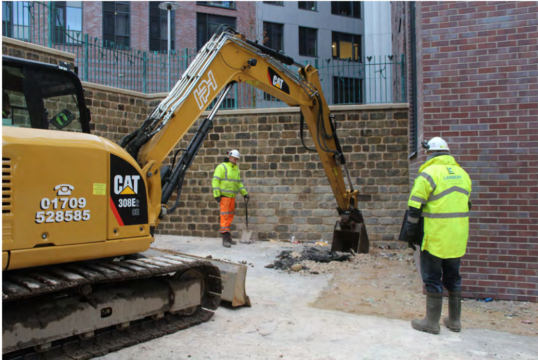
Fig. 3.5 - Removal of tarmac at location of Test Pit 3
