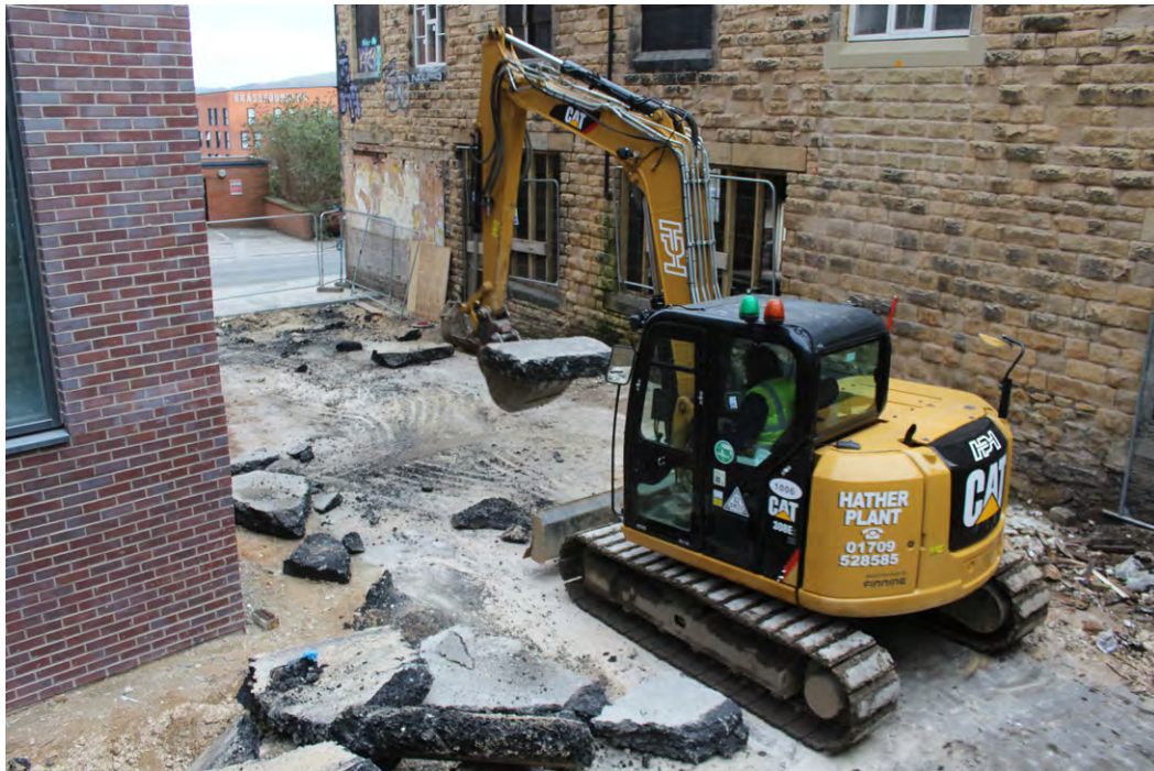
Fig. 3.2 - Removal of existing tarmac surface
