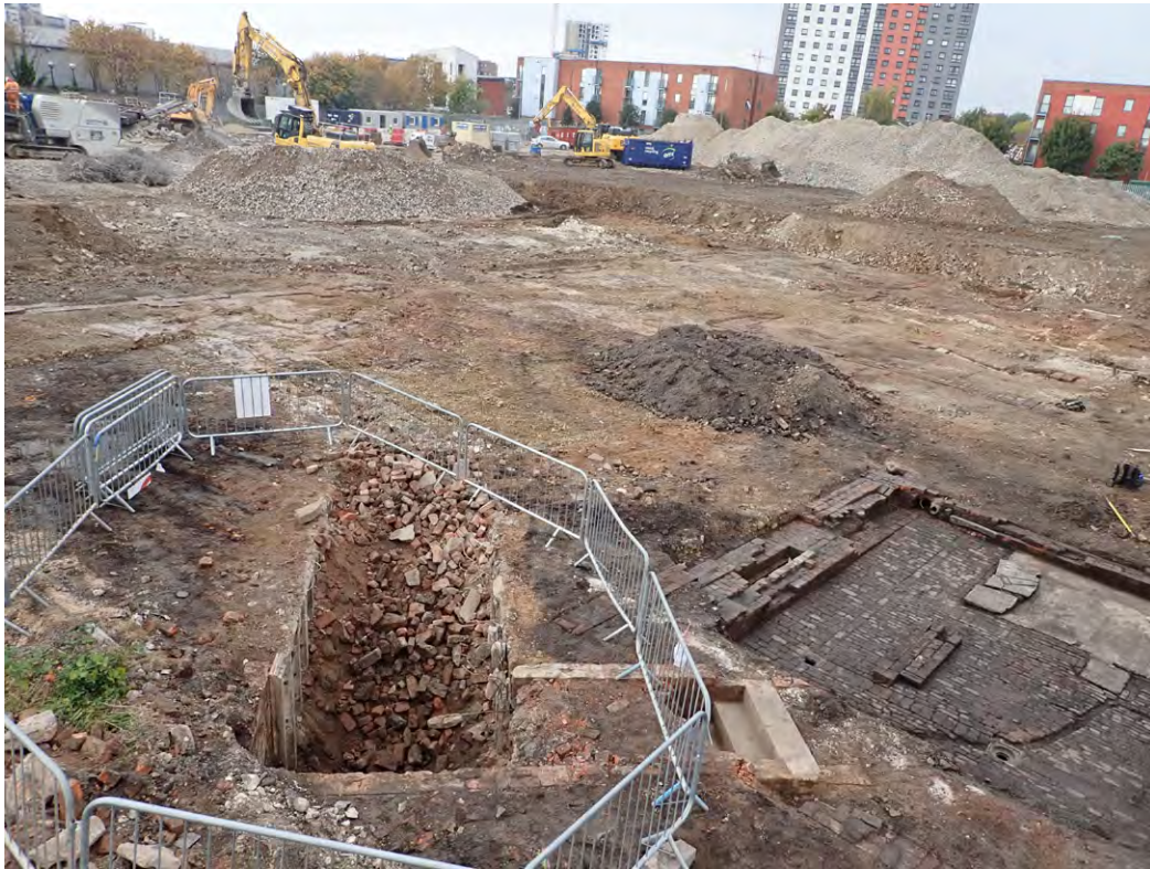
Fig. 6.1 - General view of site, looking west
