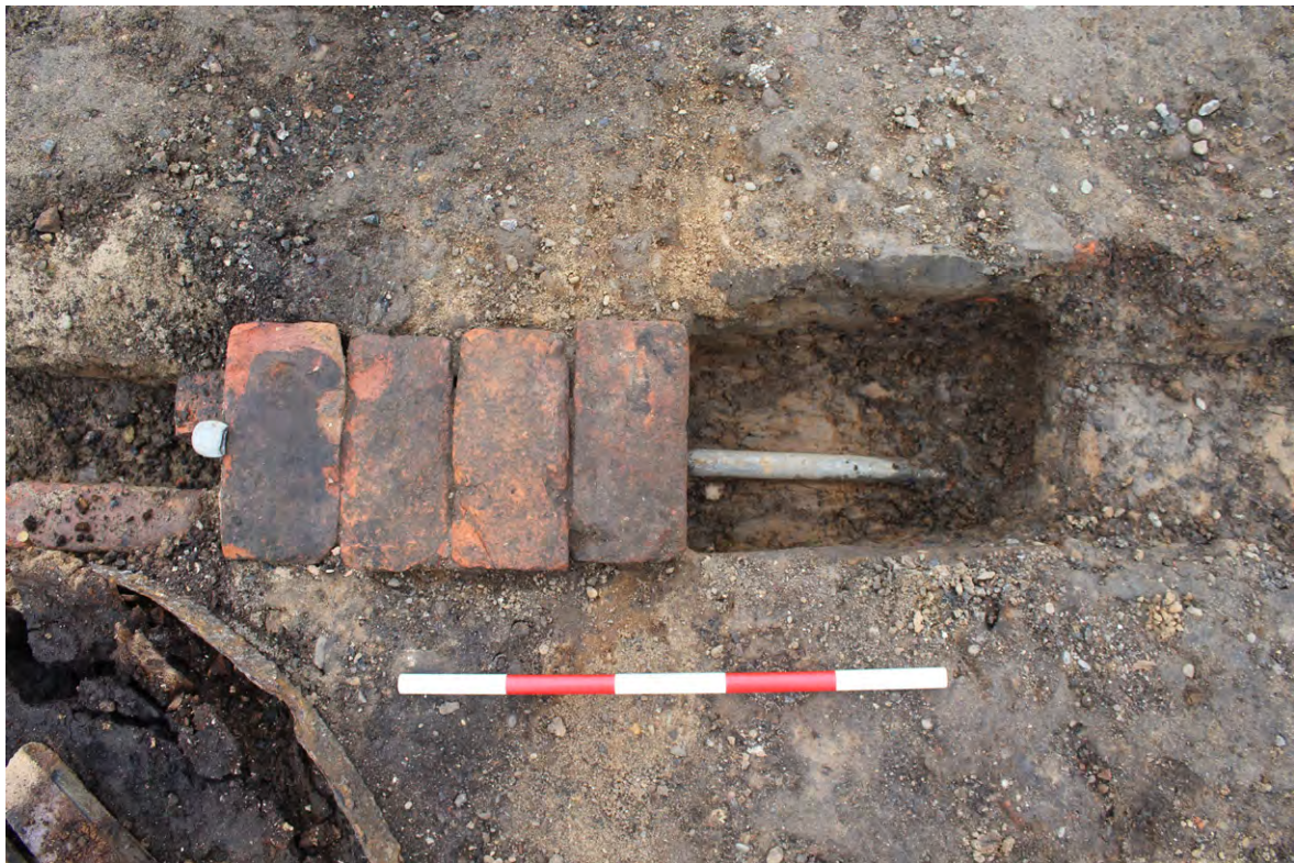
Fig. 6.22 - Brick capping 106, over lead pipe in trench 110
