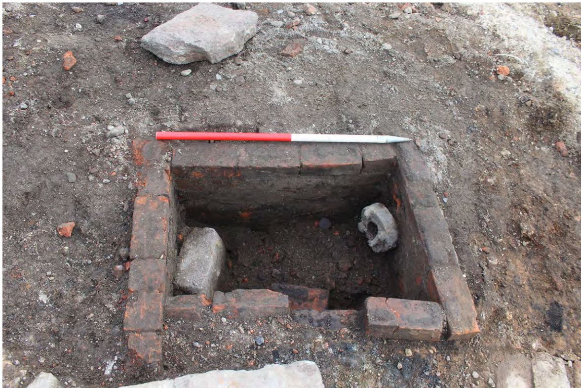
Fig. 6.24 - Brick built inspection chamber 125, looking south
