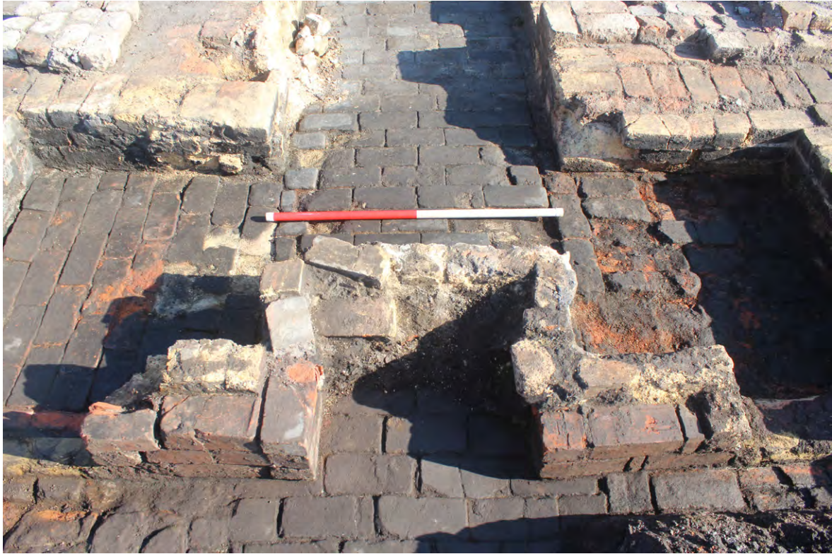
Fig. 6.45 - Wall 130 showing alcove for blow down valve, looking north-east
