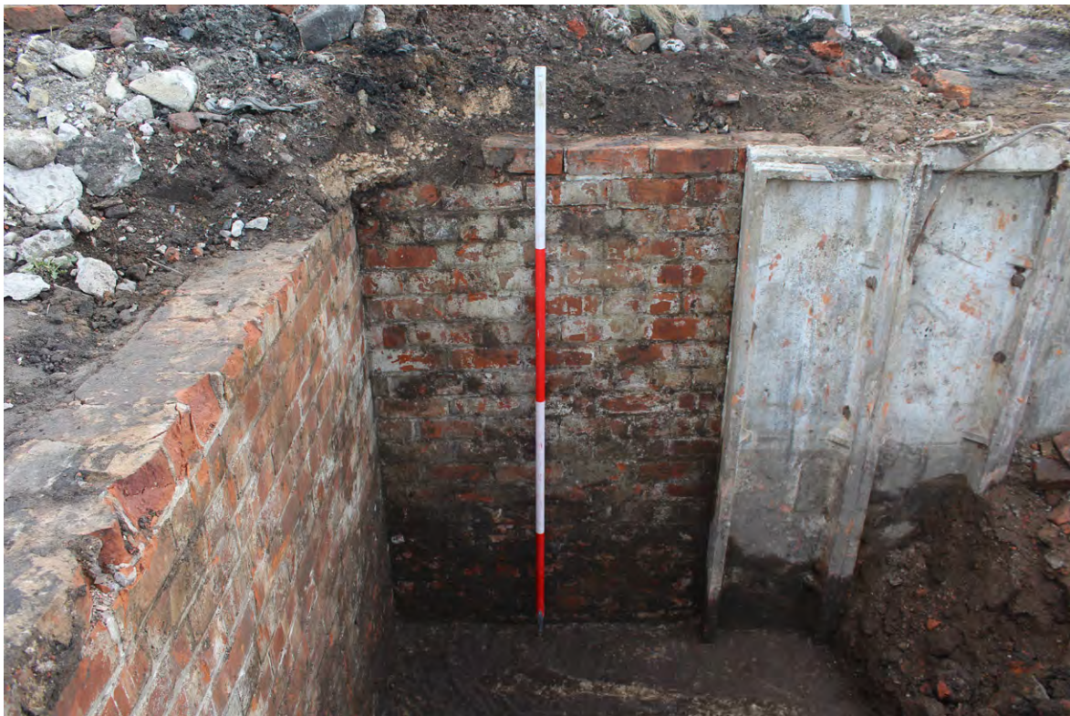
Fig. 6.4 - Construction detail at base of steps at south-eastern entrance of air raid shelter, looking south
