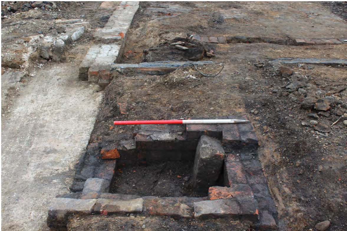
Fig. 6.17 - Brick built inspection chamber 120, looking south-east
