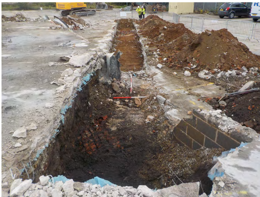
Fig. 4.2 - Trench 2 looking south-east
