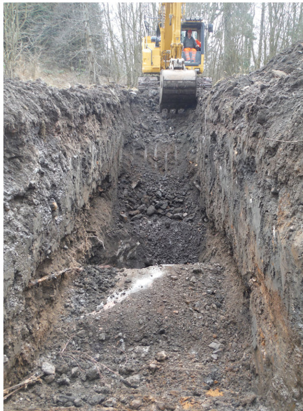
Fig. 6 - South-end of trench 3 with parallel walls 3006 in foreground
