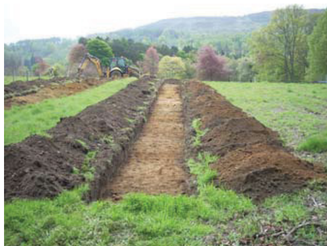
Fig. 4 Trench 2 from the NW
