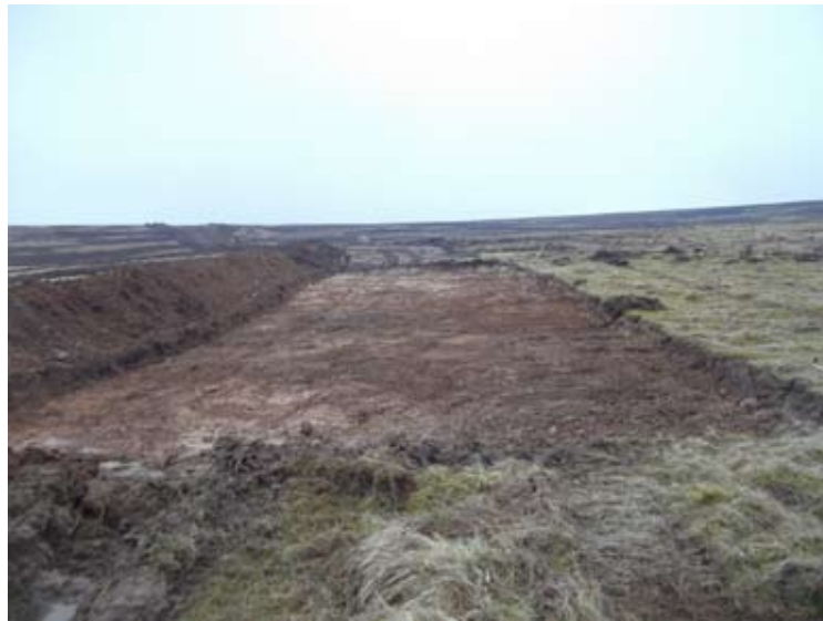
Fig 6: New road line between Dye Water crossing and chainage 7600
