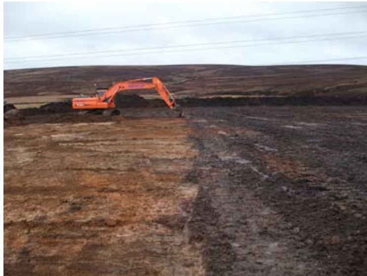
Fig 5: Topsoil stripping at substation
