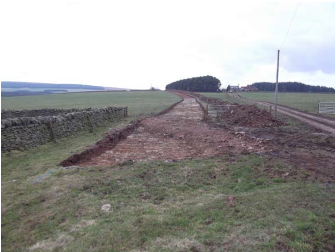
Fig 3: New road line from chainage 2600, looking north
