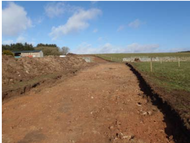
Fig 4: New road line by-passing Wedderlie Farm, chainage 1600 looking north
