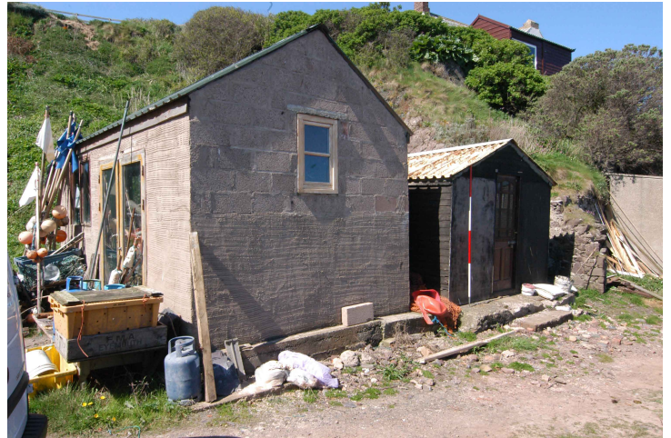
Plate 23: Fisherman's Sheds Nos. 9 & 10, east-facing elevation
