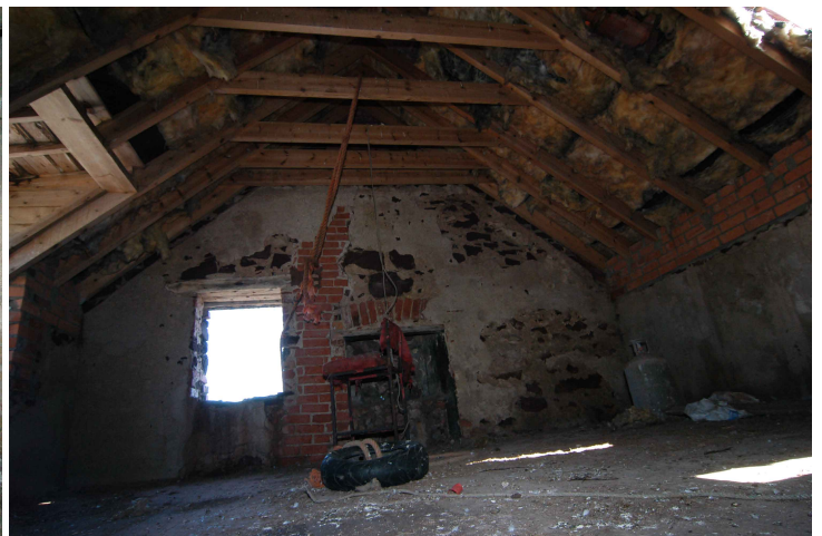
Plate 17: Building 3, Room 3 first floor interior, west-facing gable wall with fireplace
