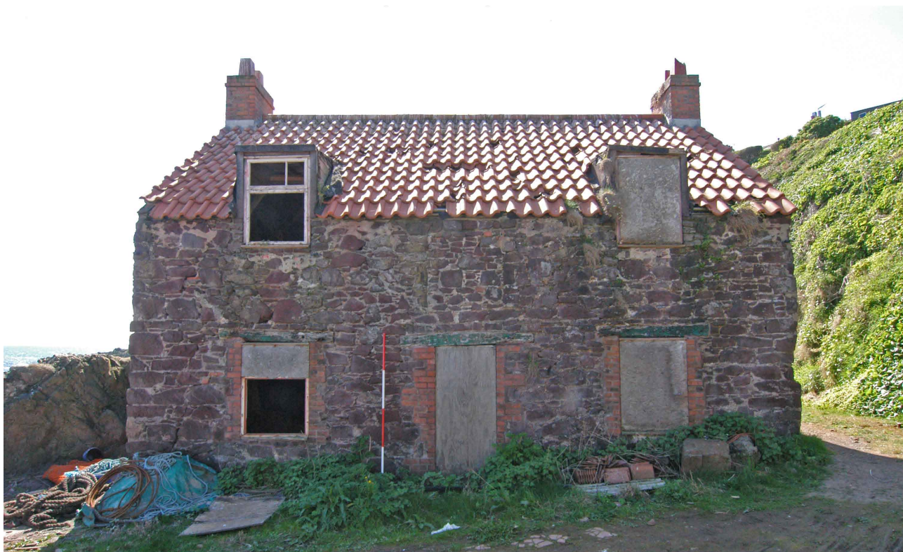
Plate 10: Building 3, Rosecroft Cottage, North-facing elevation
