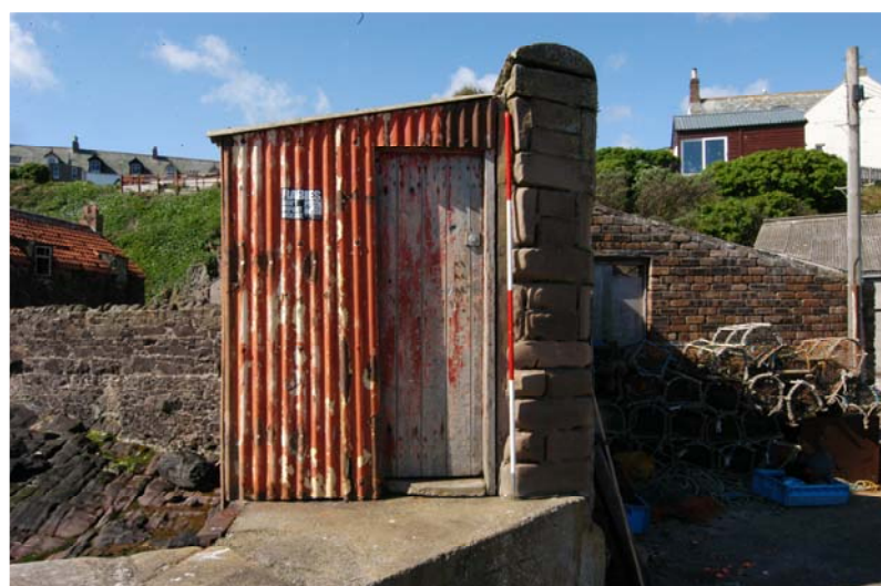
Plate 3: Building 1, Fisherman's toilet, east-facing elevation
