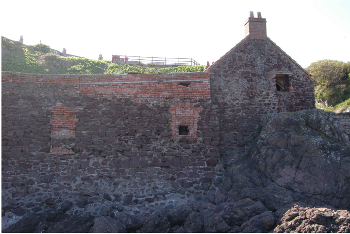
Plate 12: Building 3, East-facing gable and adjoining Building 4 and seawall
