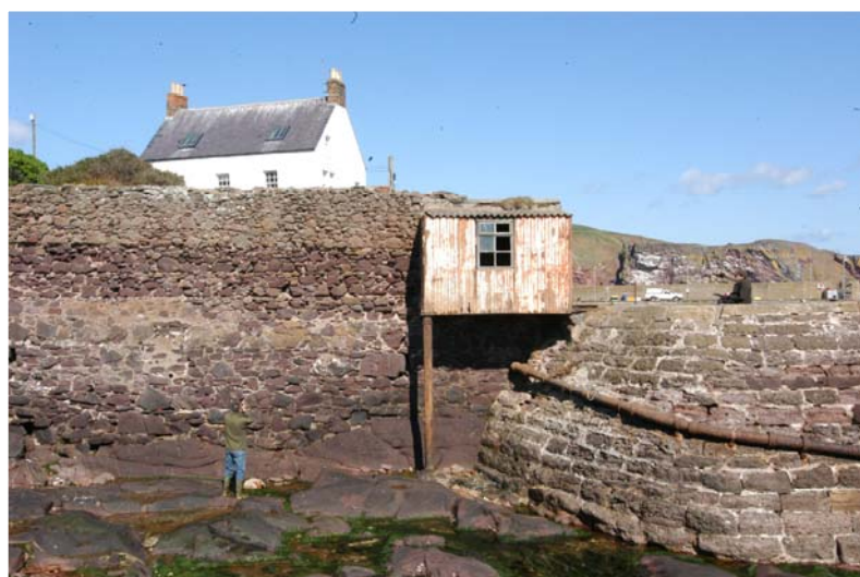
Plate 4: Building 1 Fisherman's toilets, south-facing elevation
