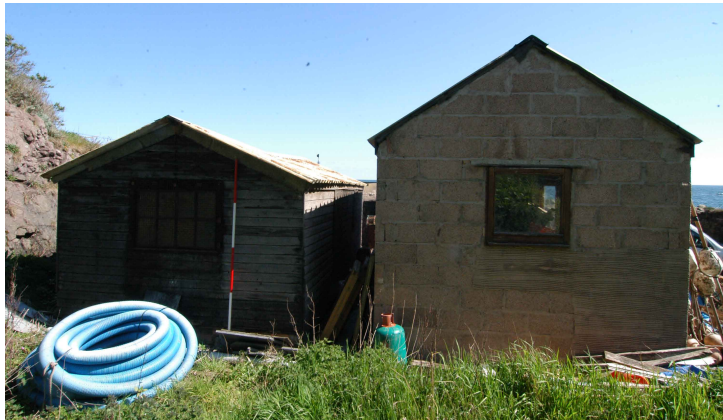
Plate 24: Fisherman's Sheds Nos. 9 & 10, west-facing elevation
