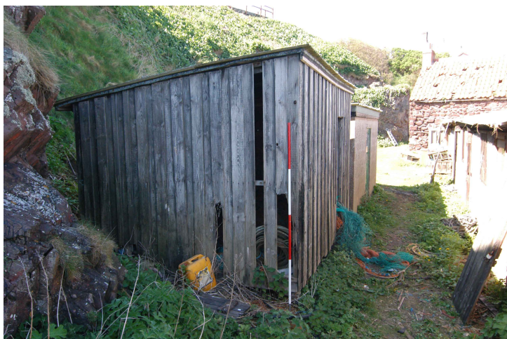
Plate 26: Fisherman's Shed No. 12, South-east corner
