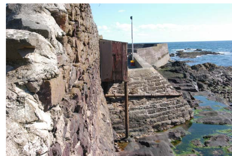
Plate 5: Building 1, Fisherman's toilet, east-facing elevation
