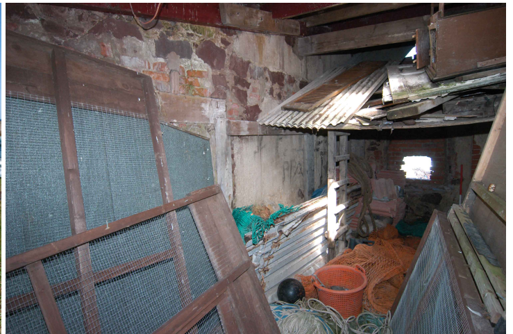
Plate 21: Building 4, Fisherman's Shed, interior of shed No 8
