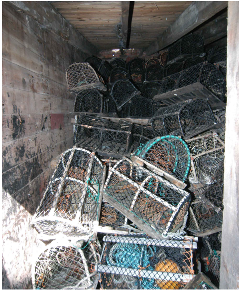
Plate 22: Building 4, Fisherman's Shed, interior of shed No 2
