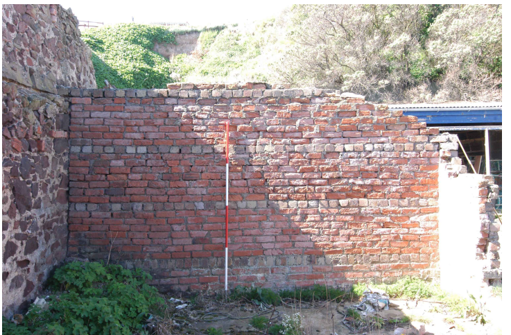
Plate 9: Building 2 Interior east-facing gable
