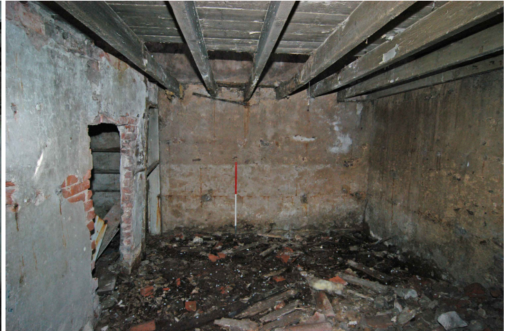
Plate 15: Building 3, Room 2 interior north-facing elevation and the stair cupboard
