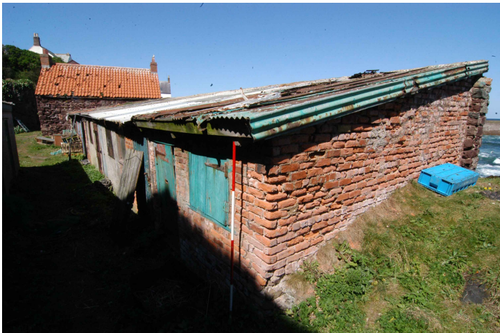
Plate 20: Building 4, Fisherman's Sheds (Nos 1-8) west-facing elevation and south-facing gable
