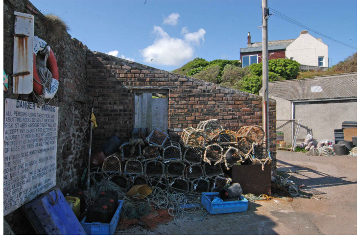
Plate 7: Building 2, former fish house, East-facing elevation
