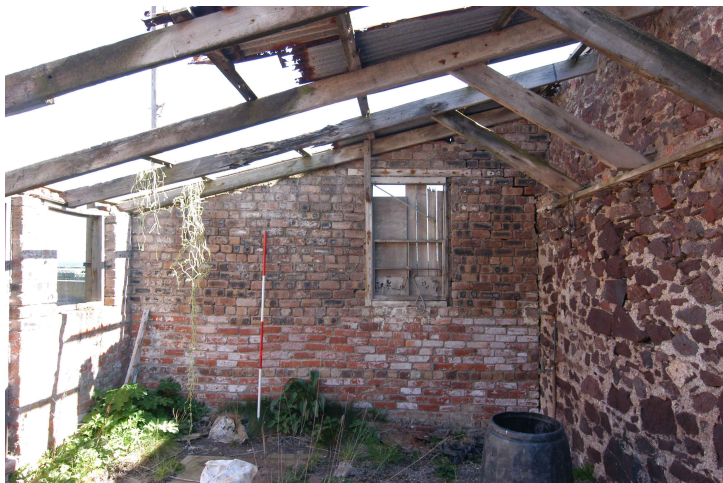
Plate 8: Building 2, former fish house, interior west-facing elevation
