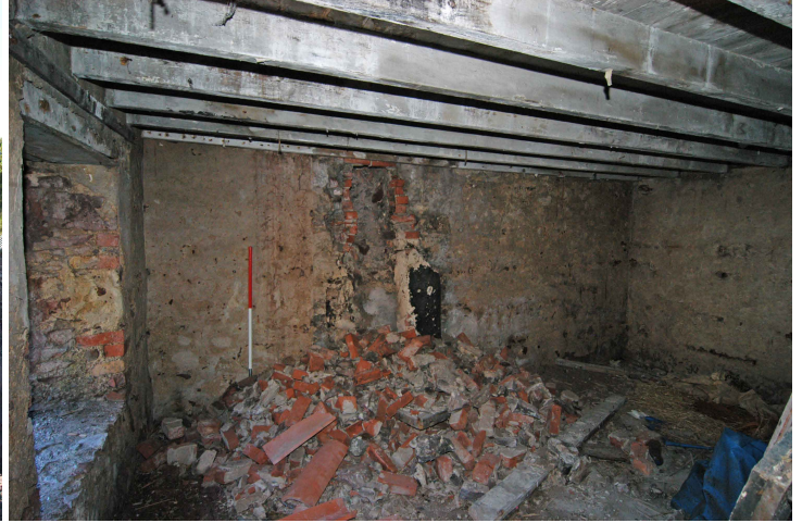
Plate 13: Building 3, Room 1 ground floor interior, west-facing elevation and floor joists
