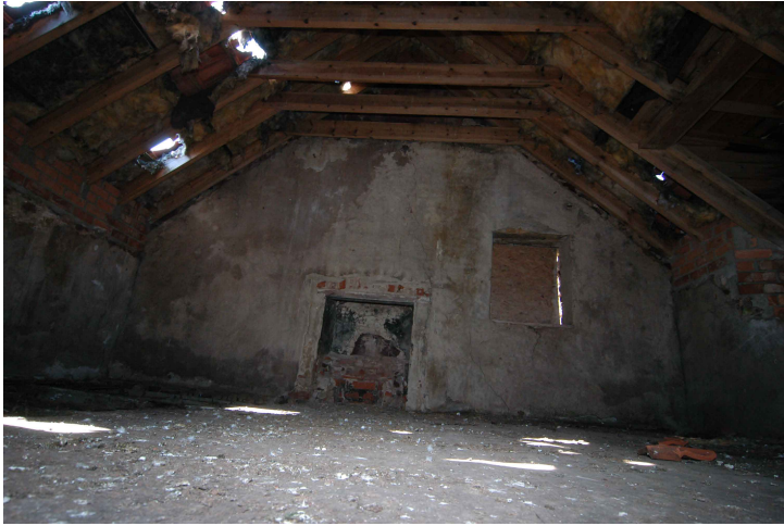
Plate 18: Building 3, Room 4 first floor interior, east-facing gable wall with fireplace
