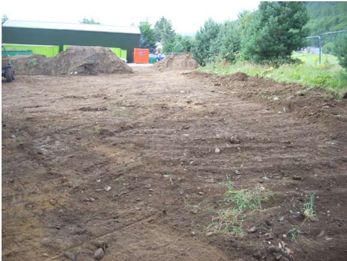
Fig 3: Temporary compound stripped of topsoil
