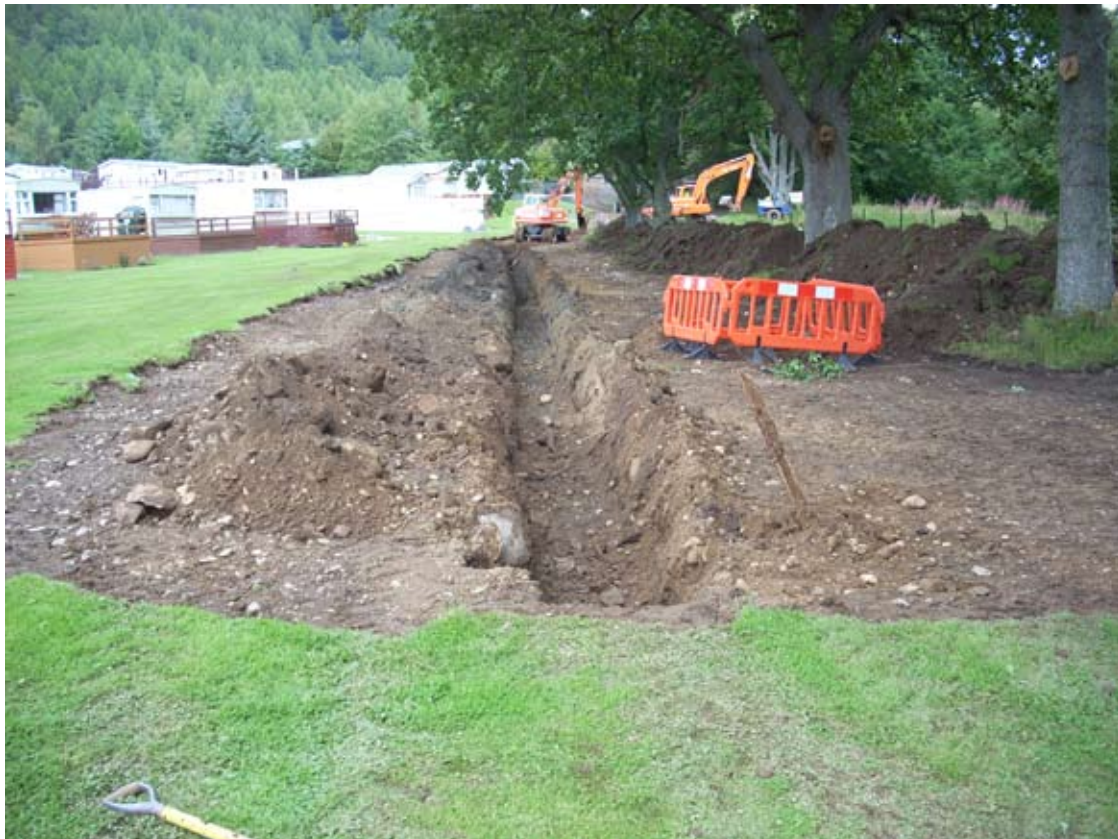
Fig 2: Pipe trench on N side of River Tay
