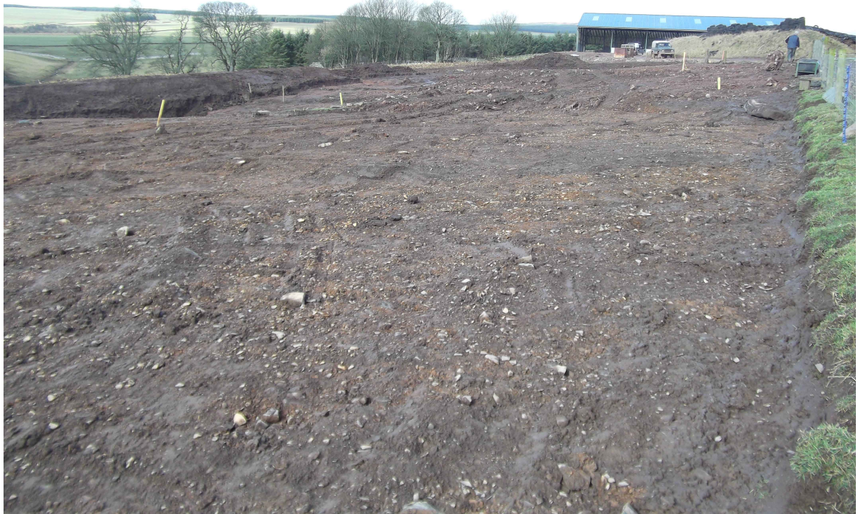
Fig. 2: General view of stripped area
