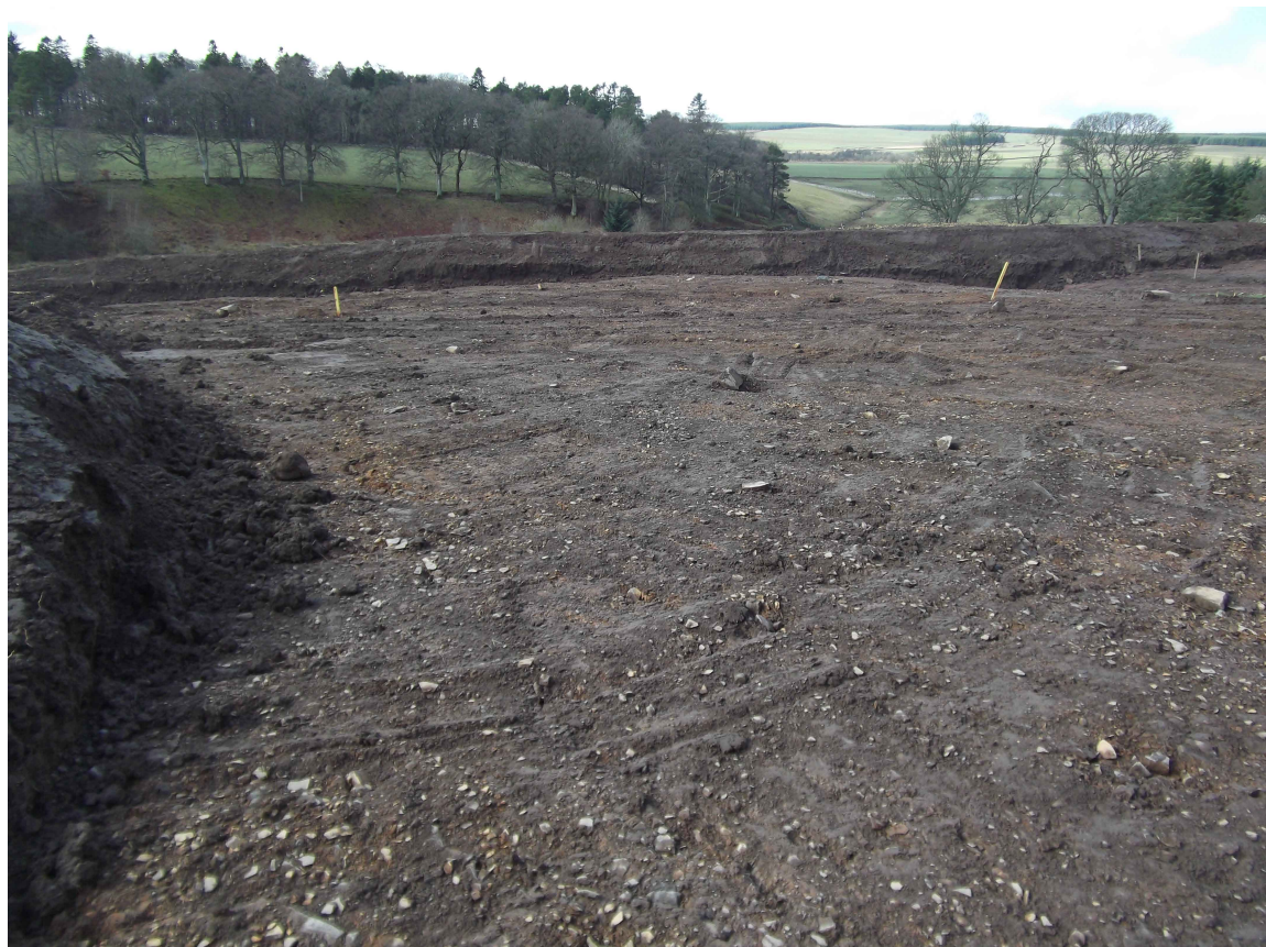
Fig. 3: General view of stripped area
