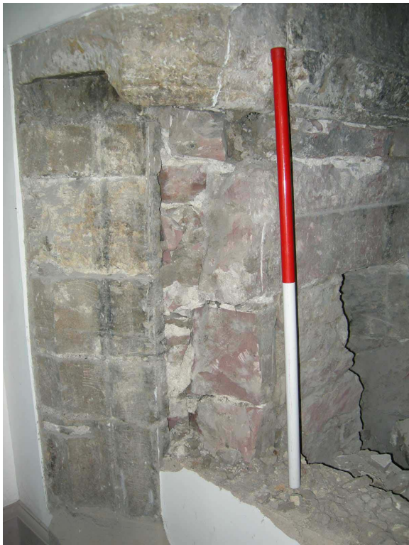
Plate 4. Unit 9, moulded ashlar stone surround on the west side of the fireplace exposed during the demolition of the strongroom
