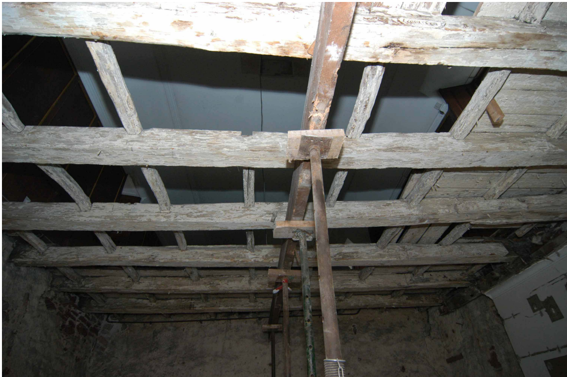
Plate 6. Unit 9, oak floor joists above the former strongroom
