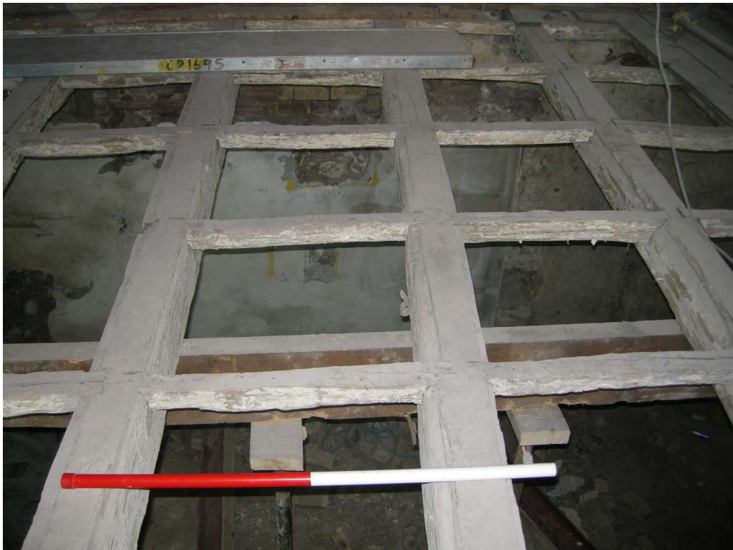
Plate 7. Unit 11, exposed floor joists following the partial removal of the Council Chamber floor
