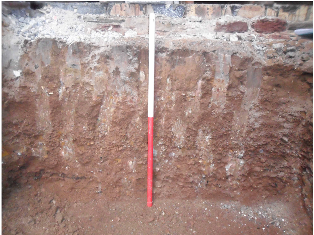
Plate 10. Exposed section on the lift shaft showing natural gravel
