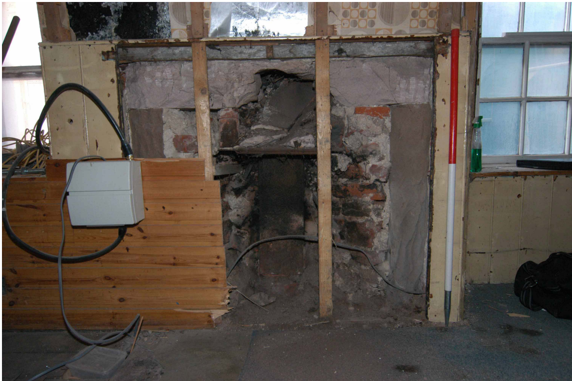
Plate 1. Unit 1, exposed fireplace on the north-facing elevation
