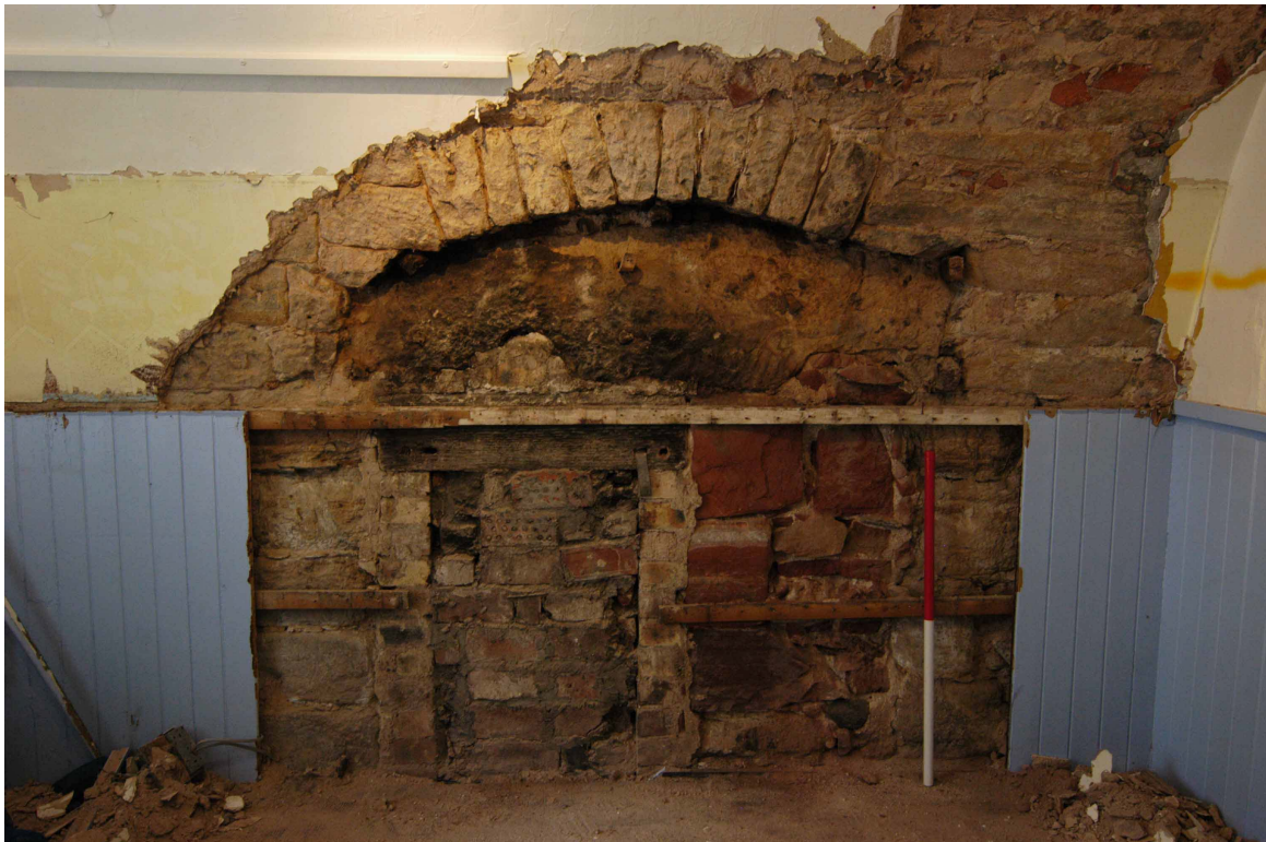
Plate 2. Unit 3, exposed blocked fireplace on the south-facing elevation
