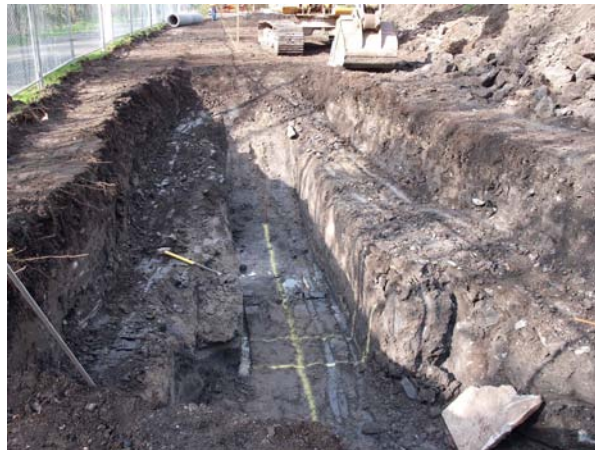
Fig.3 Post excavation shot of sewer trench
