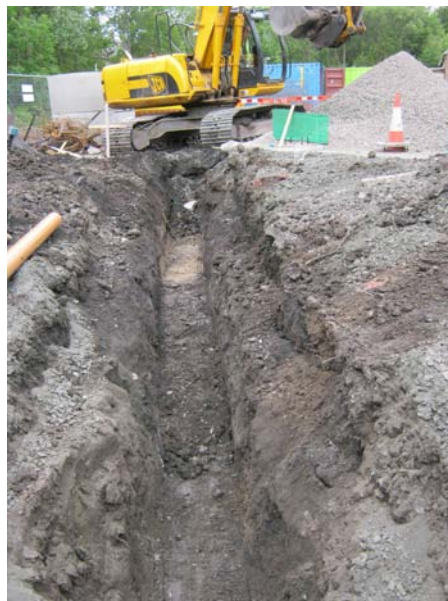
Fig.4 Post excavation shot of Trench 3
