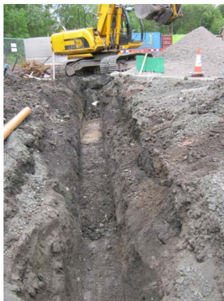
Fig.4 Post excavation shot of Trench 3
