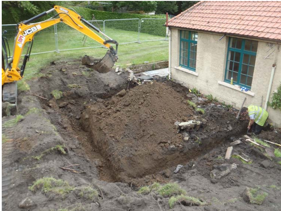
Fig. 3 General work shot of foundation trench excavation
