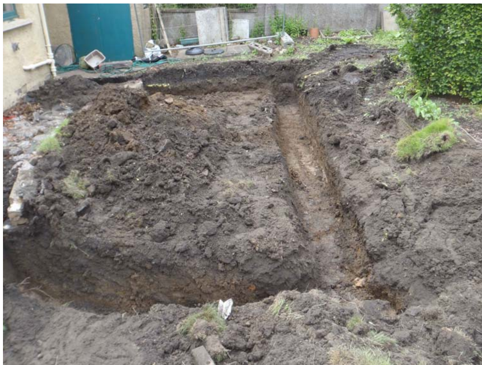
Fig. 4 View of fully excavated foundation
