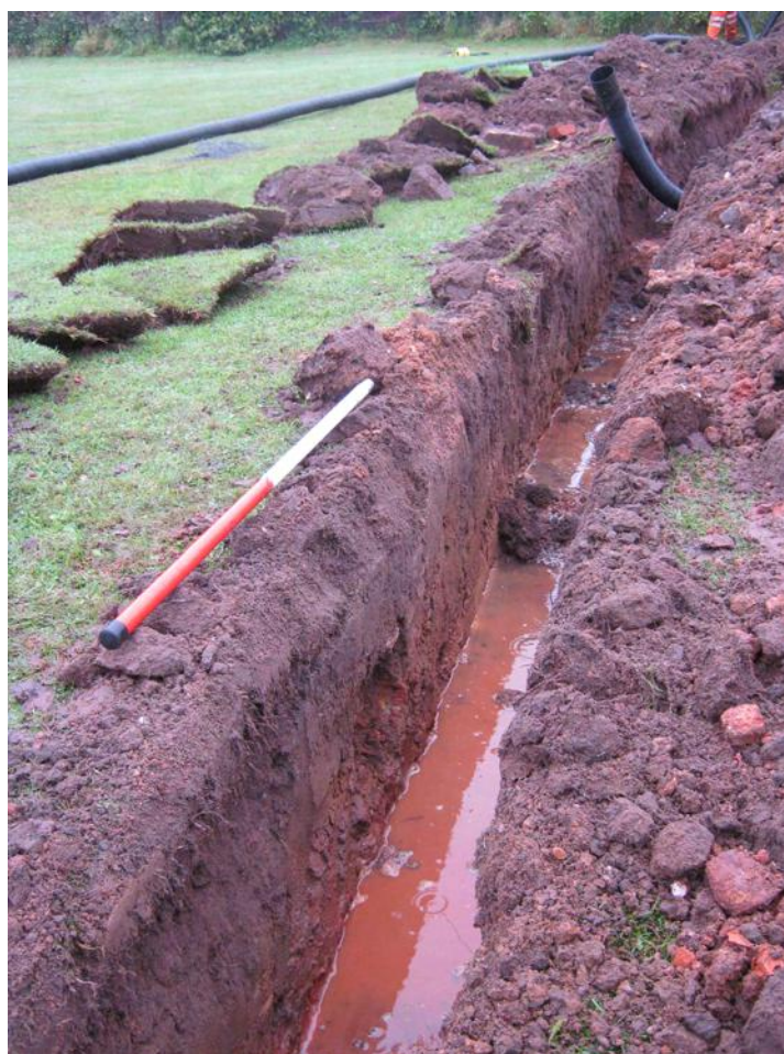
Fig. 3 - Oblique of duct trench showing topsoil overlying red sandstone
