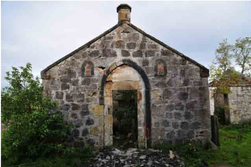
Fig 5 - Steading west range entrance from south
