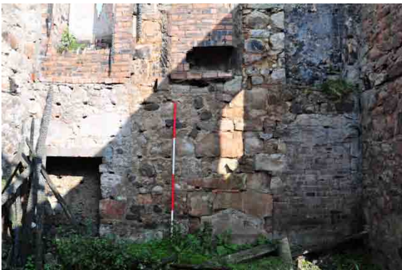
Fig 4 - House Units 7 & 14, west-facing elevation
