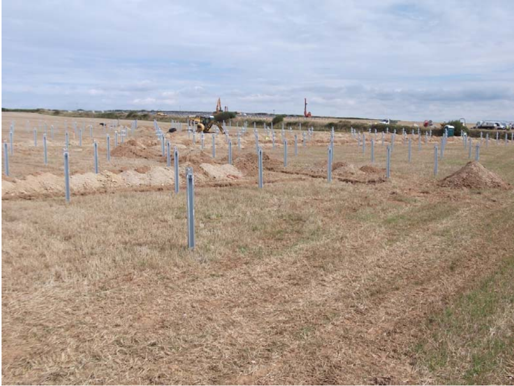
Plate1: General Site View
