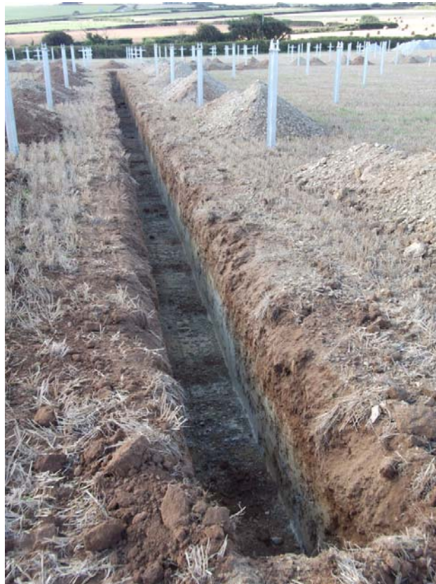
Plate 2: View of Trench in Western Field
